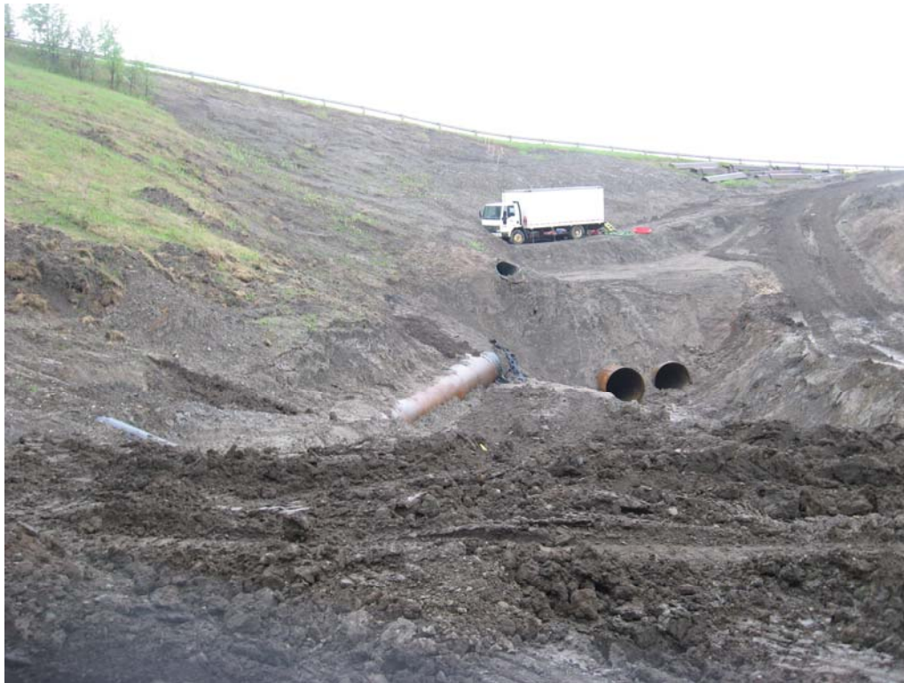
Photo 7 - View of open cut excavation at the culvert inlet, looking northwest.
