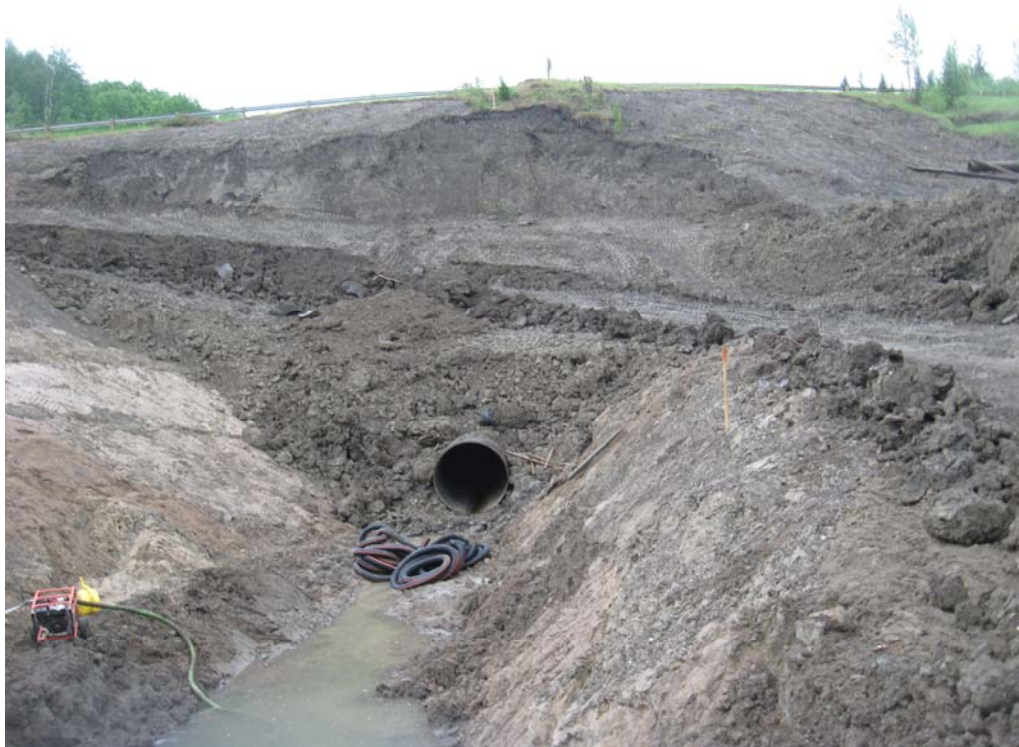
Photo 6 – View of open cut excavation at the culvert outlet, looking southeast.
