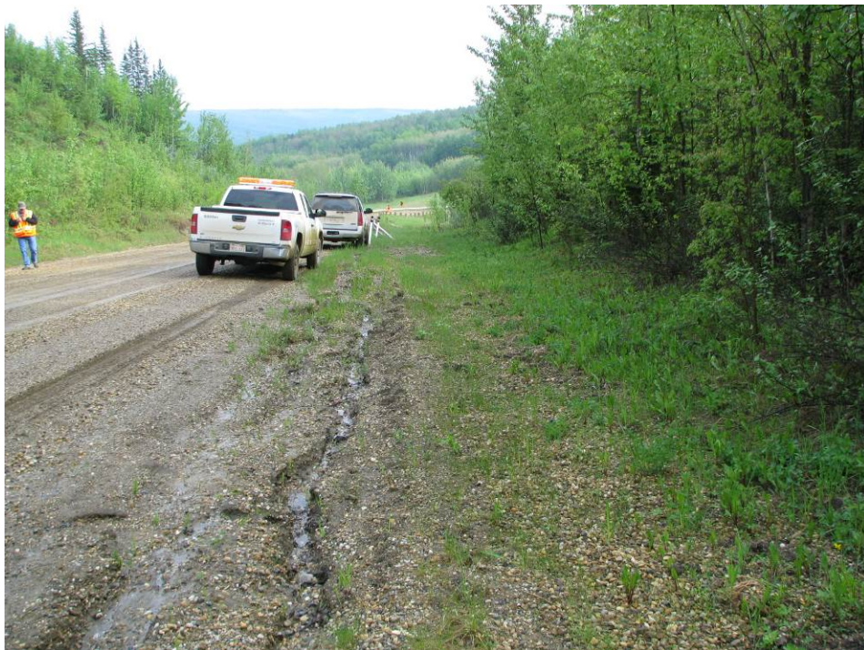
Photo 2 – Ditch erosion on the south end of the site, looking north.
