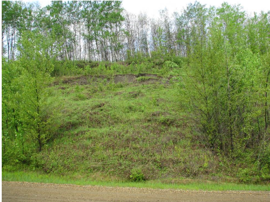
Photo 1 – Shallow back slope failures on the south end of the site, looking west.
