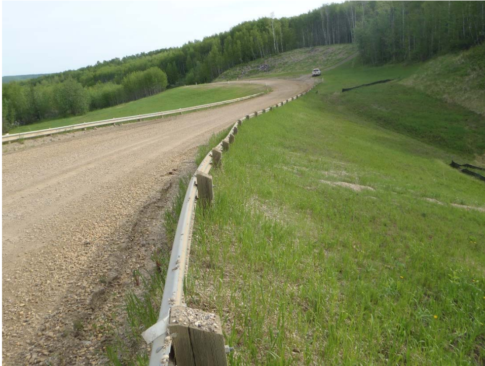
Photo 5 – Looking north along east guardrail. Note deflection in guardrail at gully.
