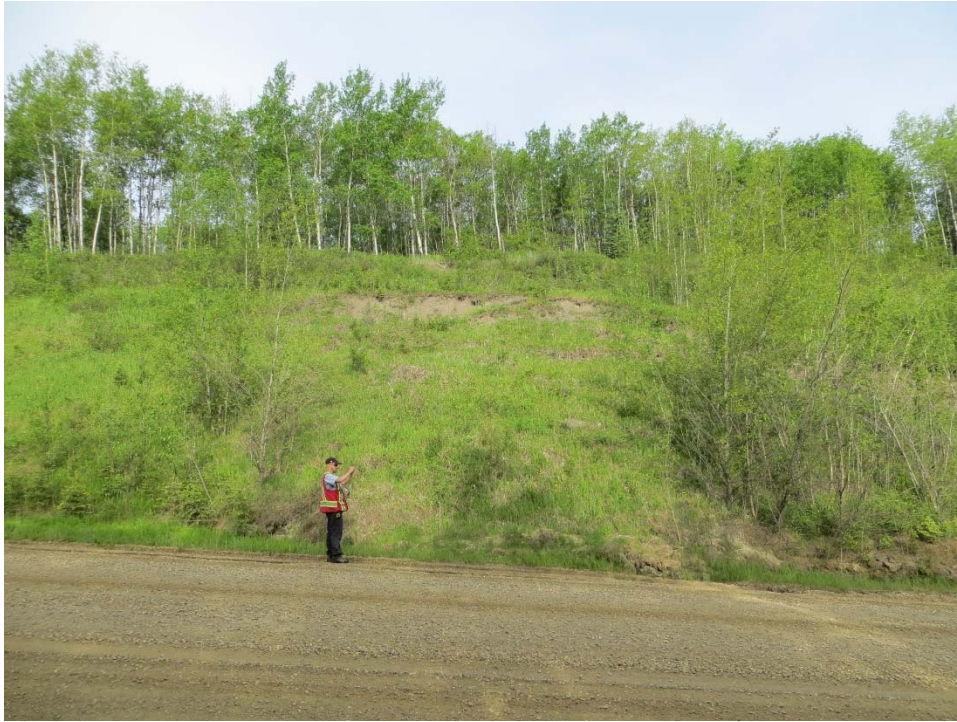
Photo 1 – Looking west at shallow west backslope failures on the south end of the site.
