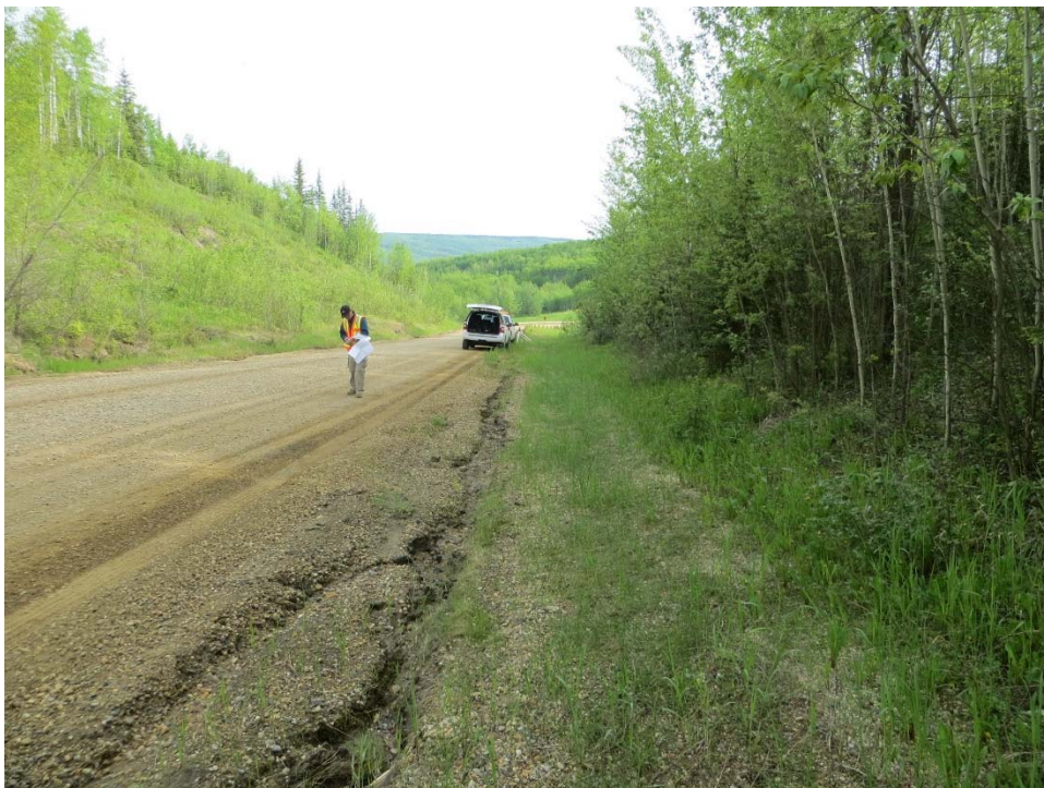
Photo 2 – Looking north at east ditch erosion at the south end of the site.
