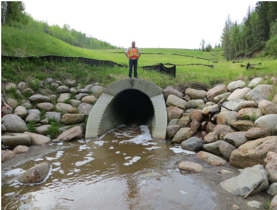
Photo 6 – Looking southeast at culvert outlet. Note erosion in riprap on right side of the culvert.
