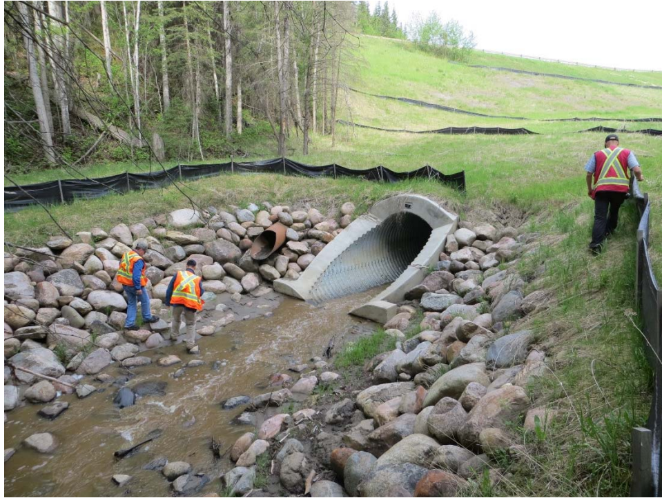
Photo 7 – Looking northwest at culvert inlet. Note erosion to right of culvert above the riprap.
