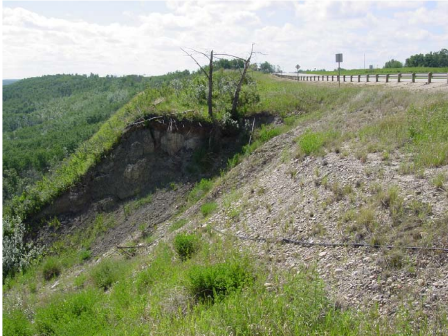
PHOTO 5: Slide 1, showing no significant changes from last year, June 12, 2006.
