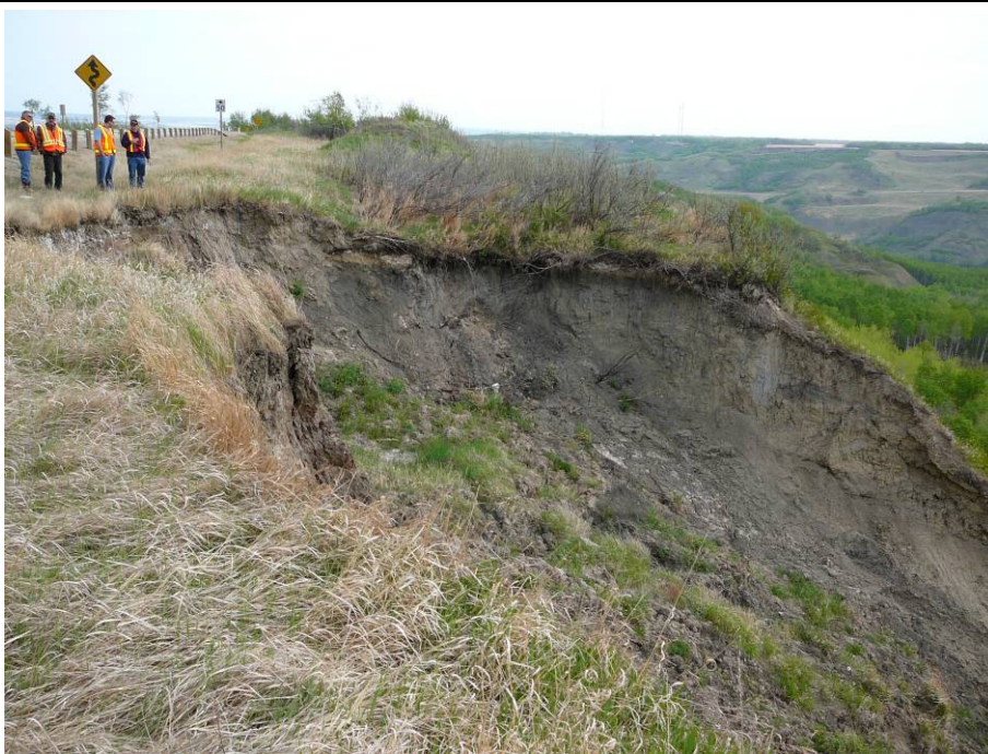
Photo 4. North end of Slide 2. There may be some fresh movement at this end of the slide, though there is some grass take on the debris at this end of the slide bowl.
