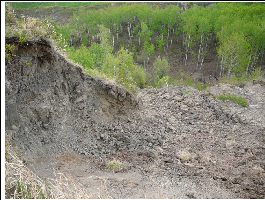
Photo 7. Slide runout for Slide 4. Note the steep, high flanks of the slide bowl.
