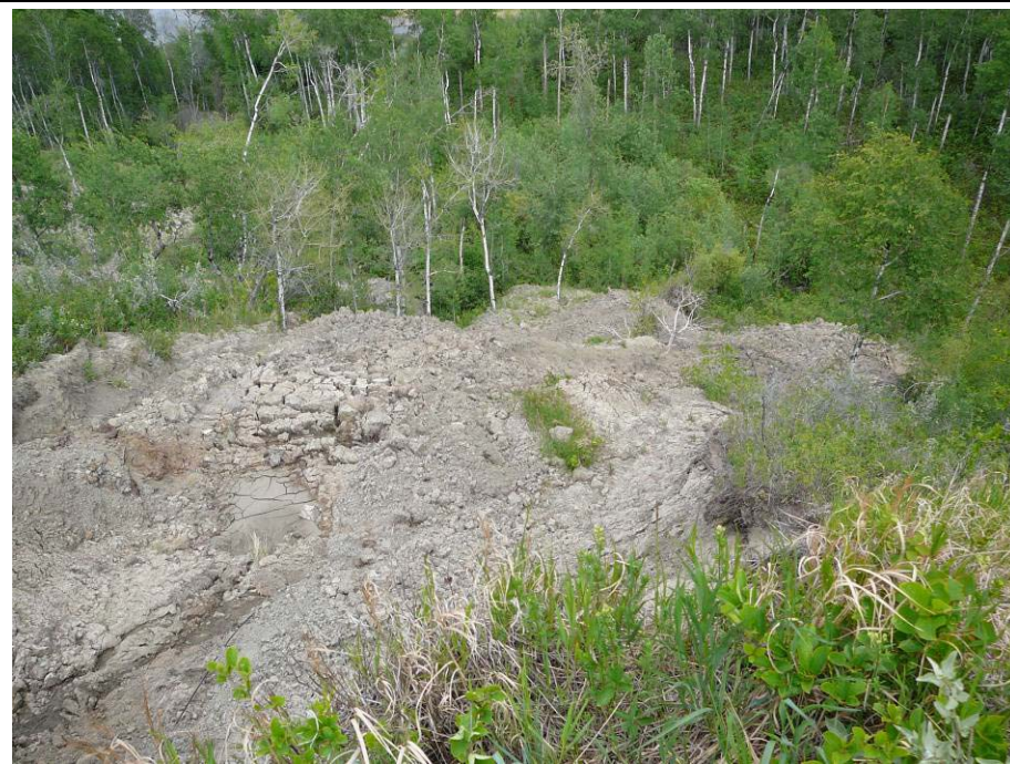
Photo 8. Looking downslope at the debris runout from Slide 4.
