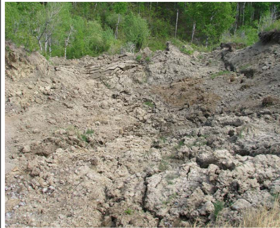
Photo 8. Looking downslope at additional debris surface flow from Slide 4.
