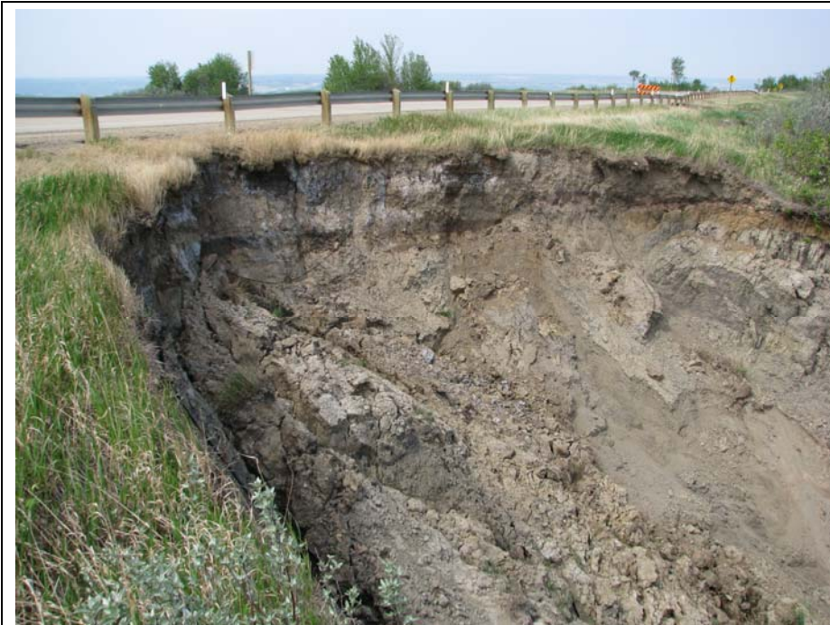
Photo 7. Looking northwards across the backscarp of Slide 4. There has been retrogression since 2010 and some movement in the slide bowl, which is now 30 m in width. The backscarp height is roughly the same as in 2010.
