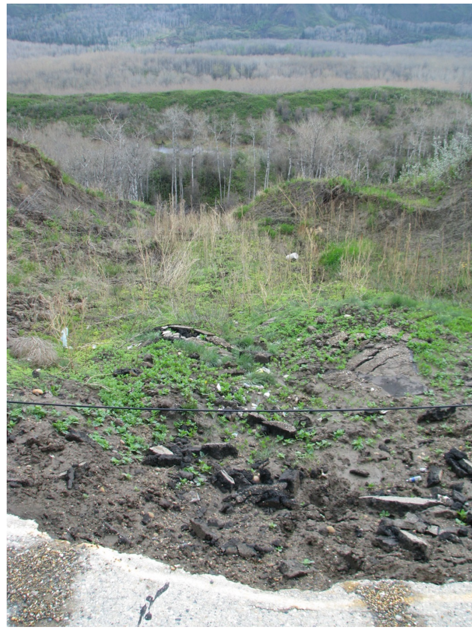
Photo 5. Slide bowl of Slide 2 – additional debris has been added since 2012. Abandoned Telus Line cable is now taught across slide bowl.
