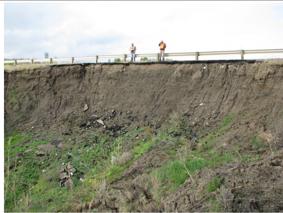
Photo 7. Looking southwest from base of Slide 3 bowl and significant accumulation of fresh landslide debris.
