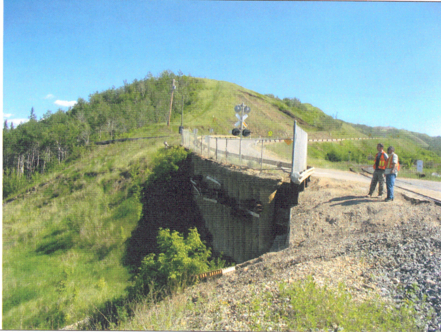
Photo 26. Pile retaining wall at the Rail slide.
