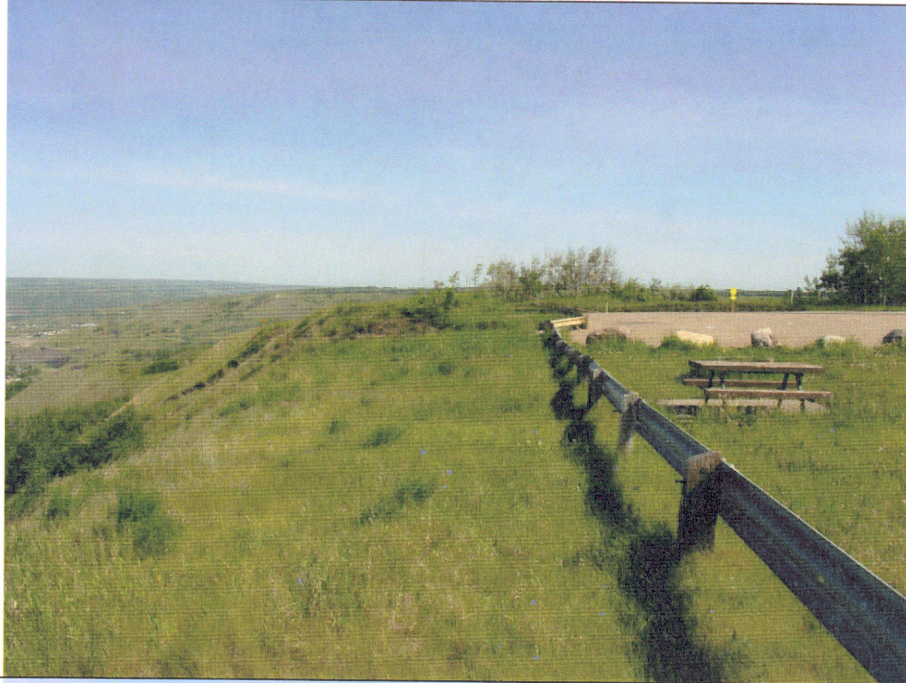
Photo 5. Looking north towards the car park area at the Lookout. Note the jog in the guardrail where the slide is encroaching on the paved area.
