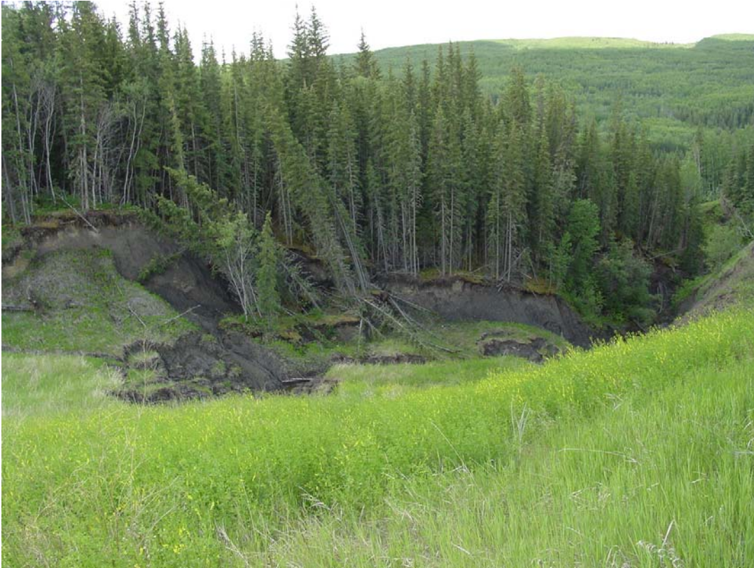
PHOTO 7: Severe slumping at and downslope of culvert extension outlet
