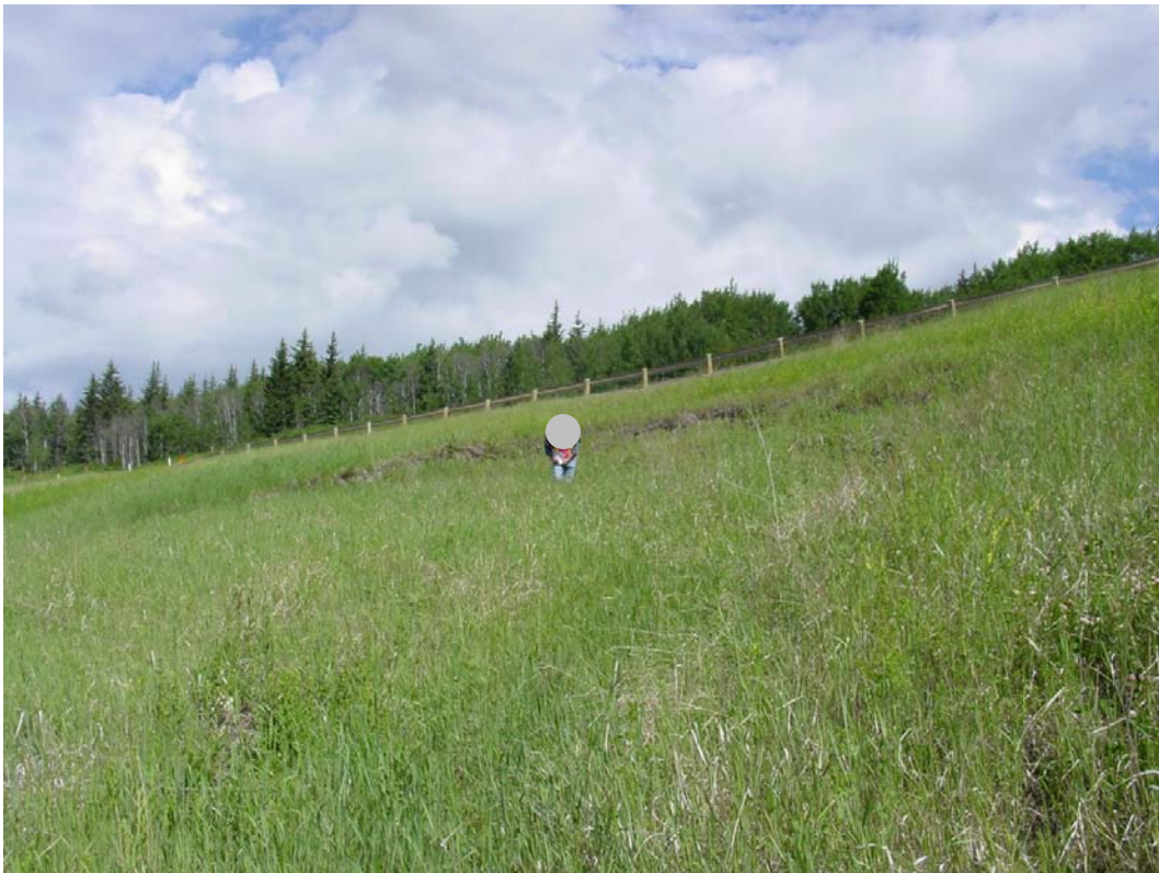
PHOTO 2: Shallow slump near top of highway sideslope
