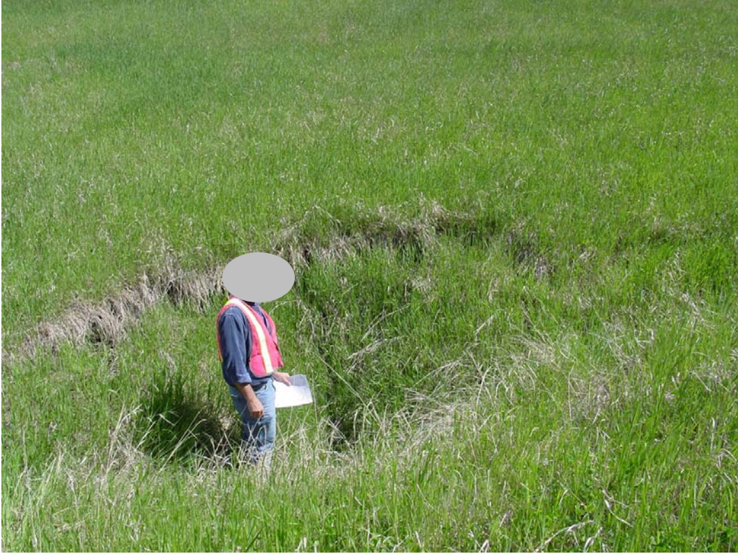
PHOTO 3: Sink hole above culvert alignment
