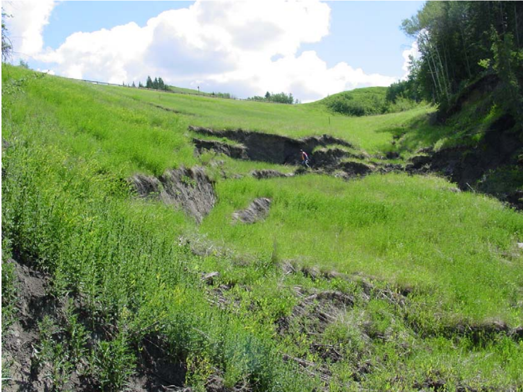
PHOTO 5: Looking northeast at severe slumping above culvert extension outlet
