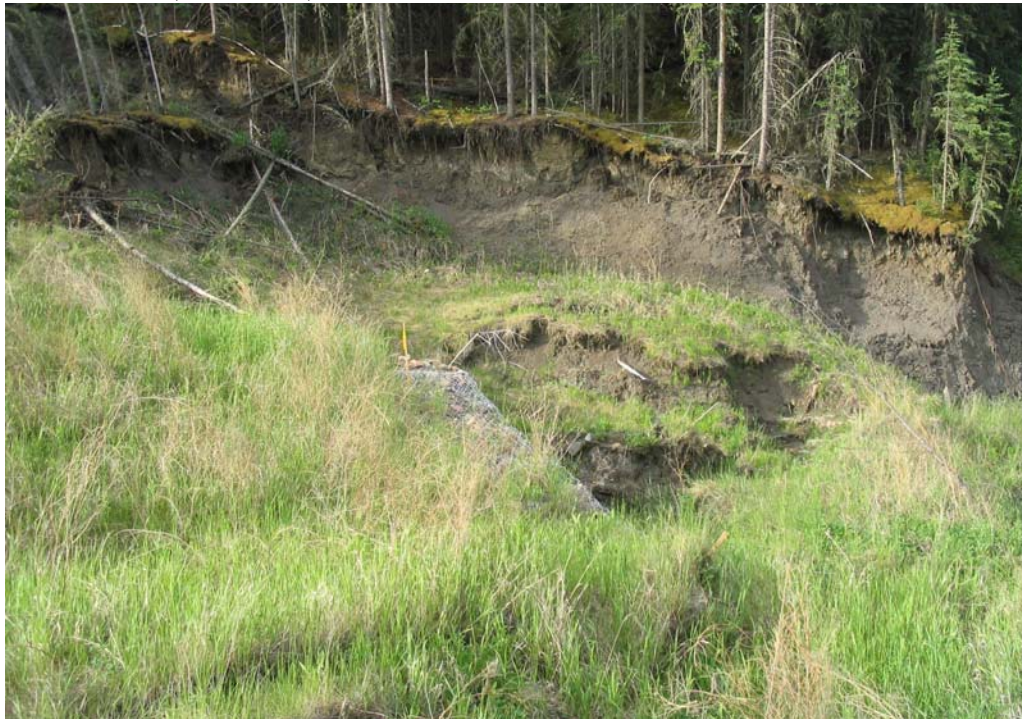
Photo 2b - Looking south across gabion outlet at severe, fresh slumping along site boundary edge, June 15, 2006.
