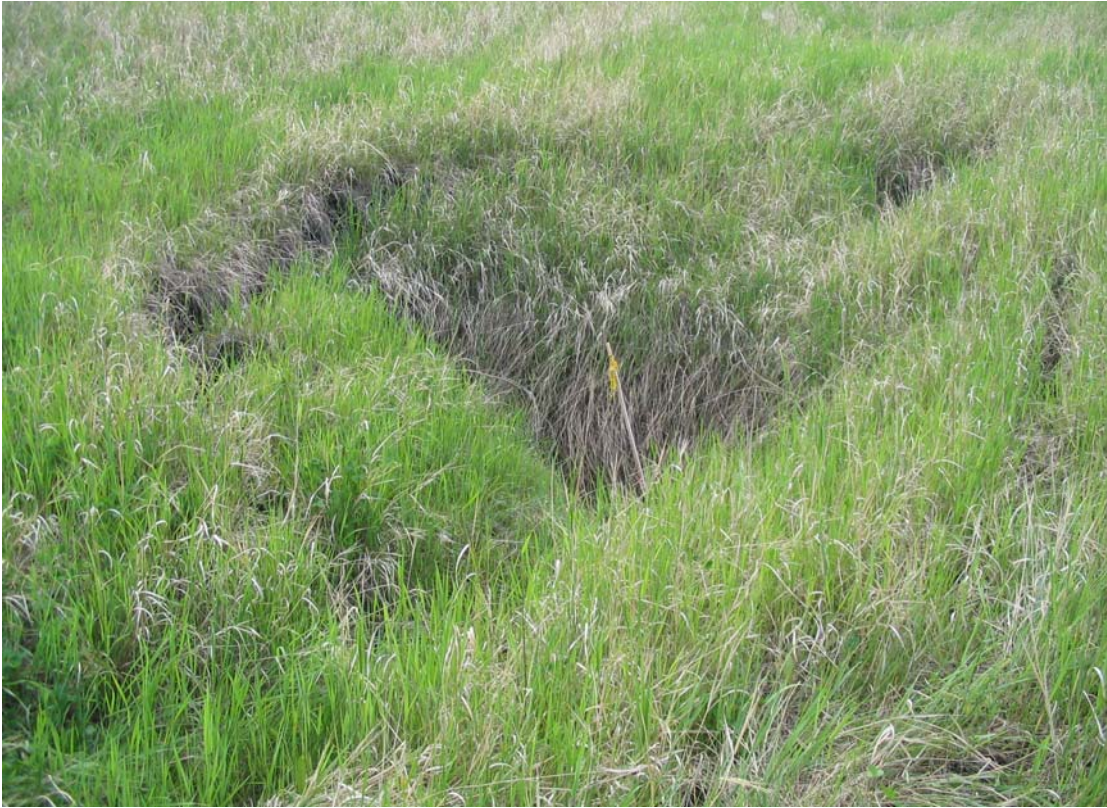
Photo 1 - Looking east at sinkhole overtop culvert alignment. Note extended cracks on south side, June 15, 2006.
