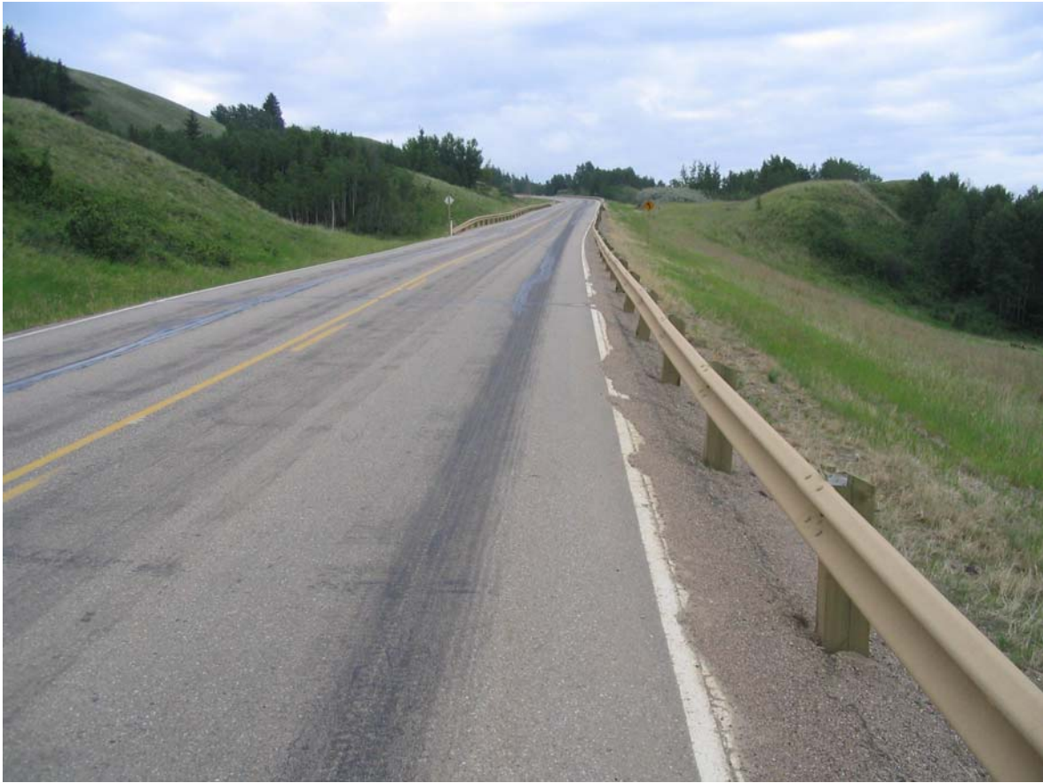
Photo 5 - Looking east along highway. Note dips in highway overtop culvert, June 15, 2006.
