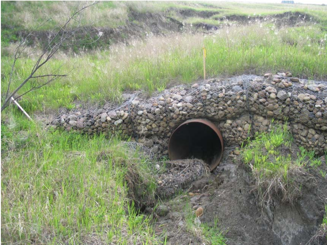
Photo 3 - Looking at culvert outlet, eroded gabions, and scarp above, June 15, 2006.
