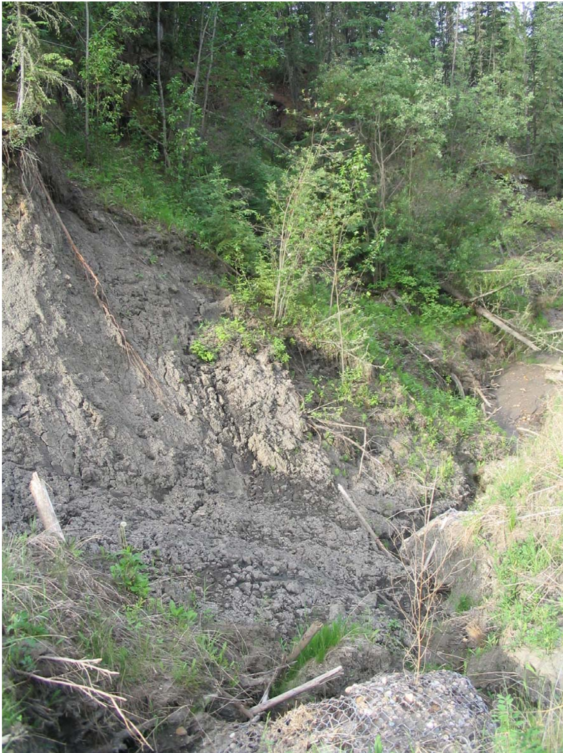
Photo 4 - Looking southwest along channel from culvert outlet at slumping and erosion June 15, 2006.
