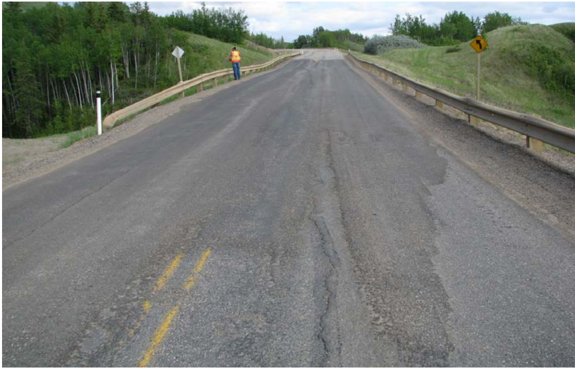
Photo 1 - Looking east along the highway over the Grimms Creek site area. Note the ACP patch and the dip in the highway.
