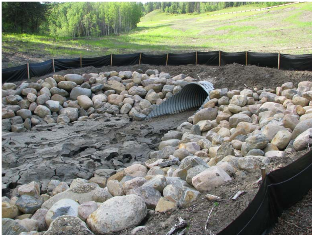
Photo 6 - Looking west across the new culvert outlet. It is about 20% full of sediment.
