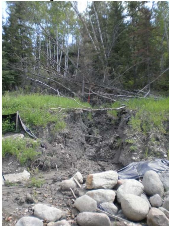
Photo 4 - Looking east at a 5 m long x 1 m deep erosion gully that has formed on the east of the channel in front of the culvert inlet.
