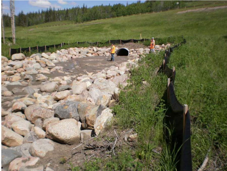
Photo 7 - Looking west across the new culvert outlet. It is about 30% full of sediment.
