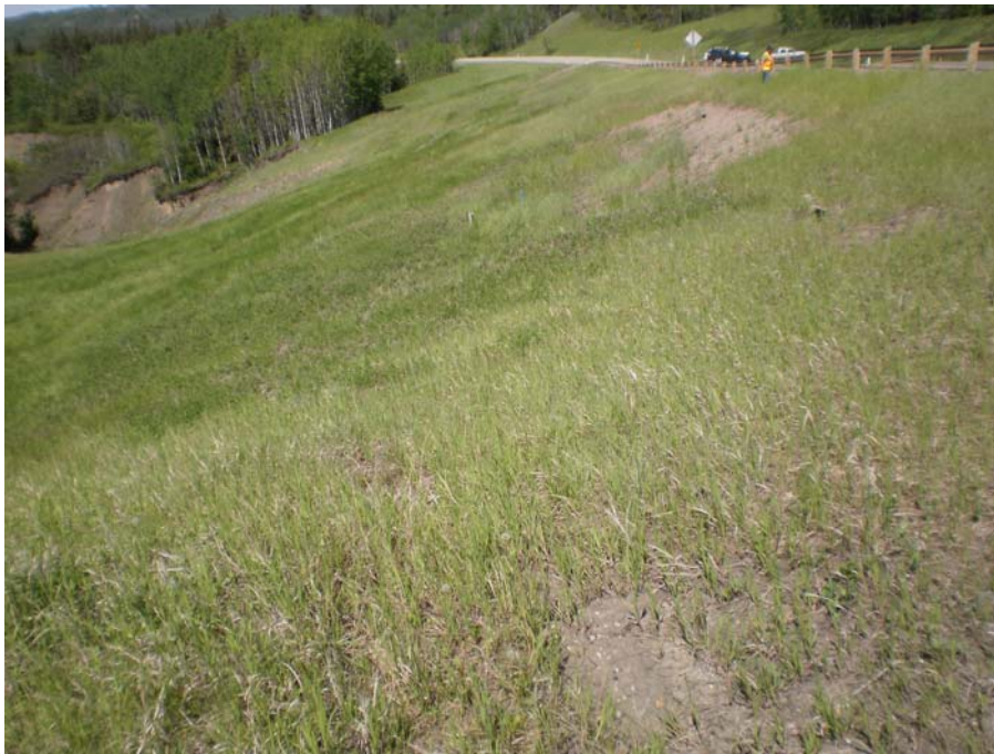
Photo 6 – Looking west across the downstream highway embankment. Note the lack of grass growth along the shallow slide scarp.
