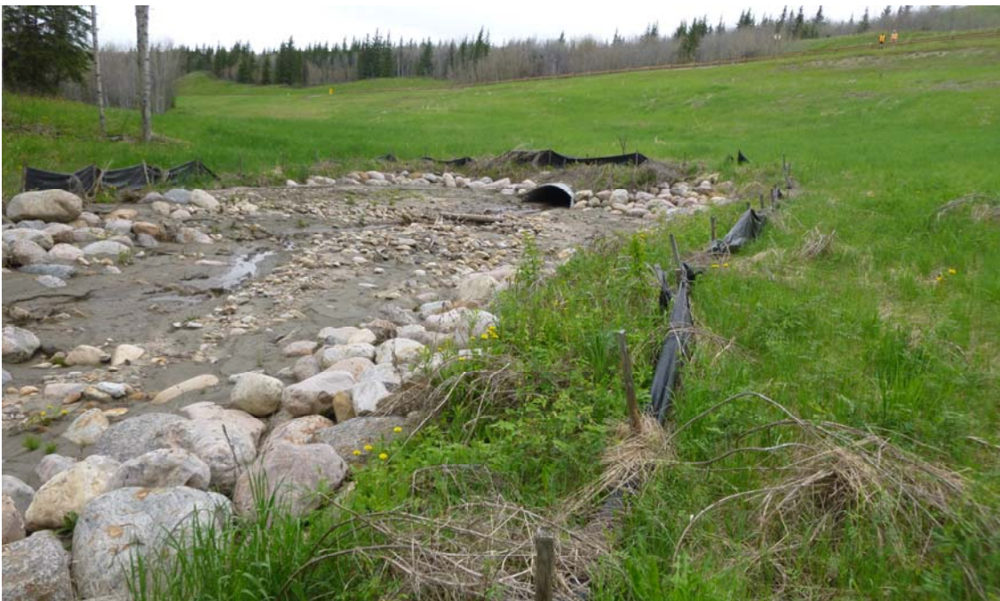
Photo 10 - Looking northwest at the new culvert outlet. It is about 60% full of sediment.
