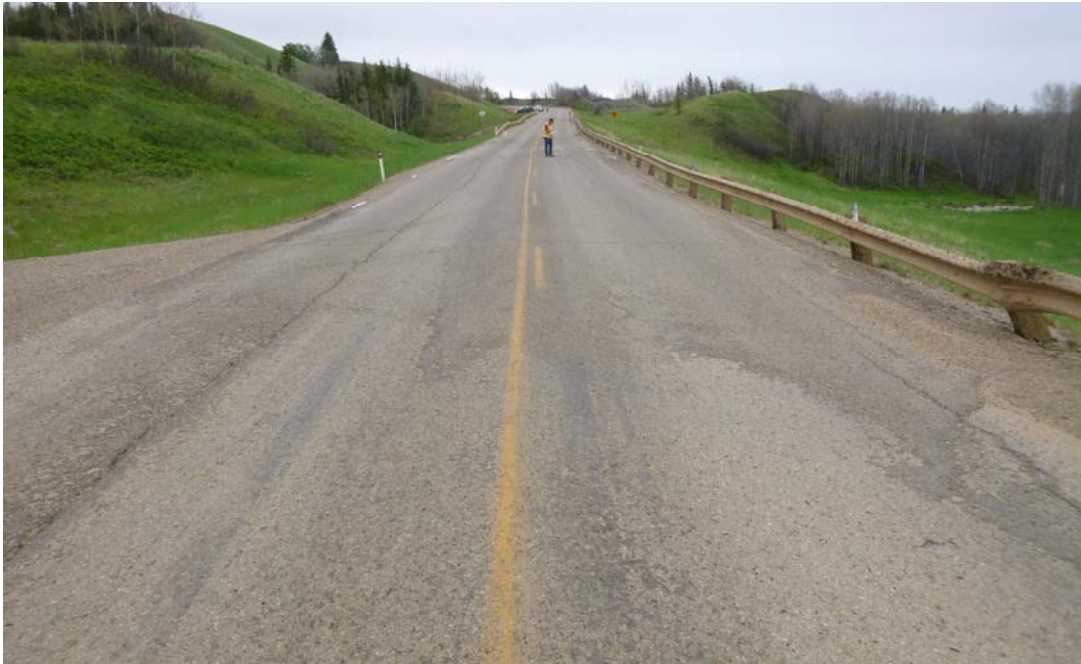
Photo 5 – Looking east along the highway over the Grimms Creek site area. Note the ACP patches, cracks and dips in the highway.
