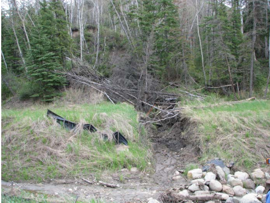
Photo 3 - Looking east at the enlarged gully and fresh erosion on the east side of the channel in front of the culvert inlet.
