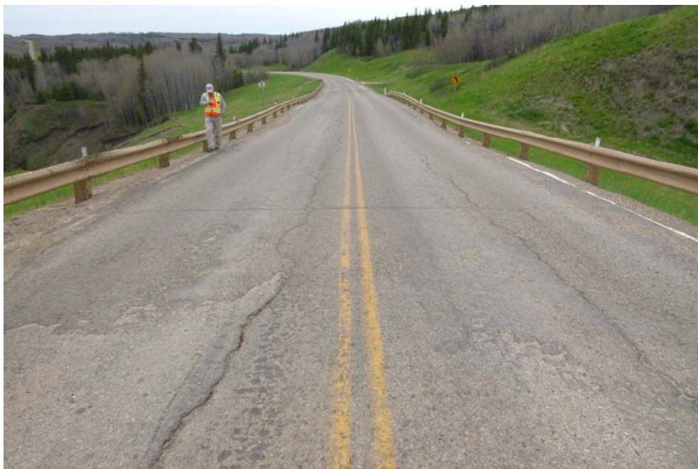
Photo 6 – Looking west along the highway. The ACP patches, cracks and dips in the highway indicate a large scarp crack may be developing along the south side of the hwy.
