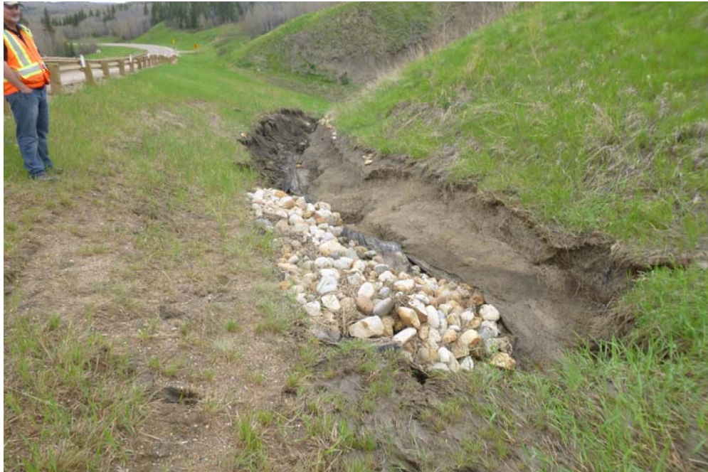
Photo 1 – Looking west at the erosion caused by highway runoff in the northeast quadrant of the site.
