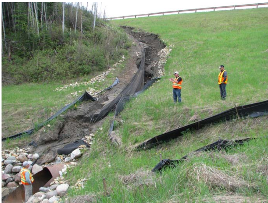
Photo 2 - Looking southeast at the culvert inlet area. Note the severe erosion that has damaged the liner installed to carry north ditch erosion – this was intact last year.
