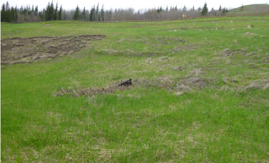
Photo 9 - Looking north at the active slumping on the south embankment slope.
