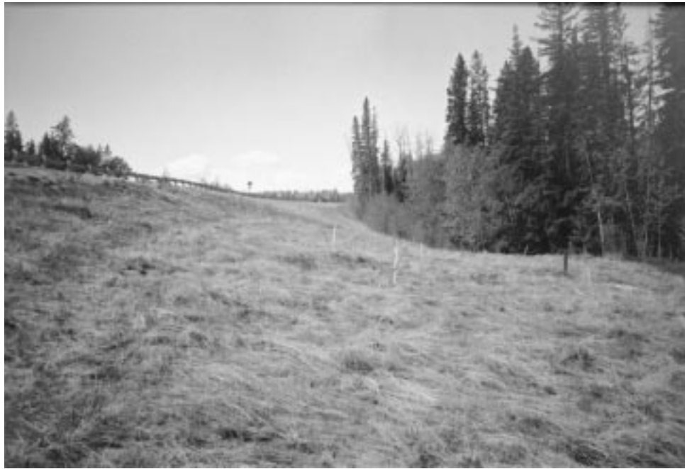
Photo 1 – General view of slope, facing west across slide area. Red casing protector on right of photo is the new SI installed in AMEC BH2 (February 2001) to replace sheared-off SI #7.
