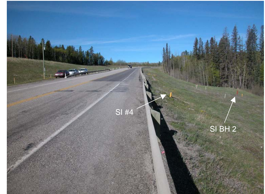
Photo S2-1 (upper left) – May 2004 – facing east across the S2-Priddis site. Note the slight bend in the guardrail visible at the far (east) end. The landslide area is visible on the slope below the road, on the left side of the photo. Photo S2-5 shows another view of the landslide area.
