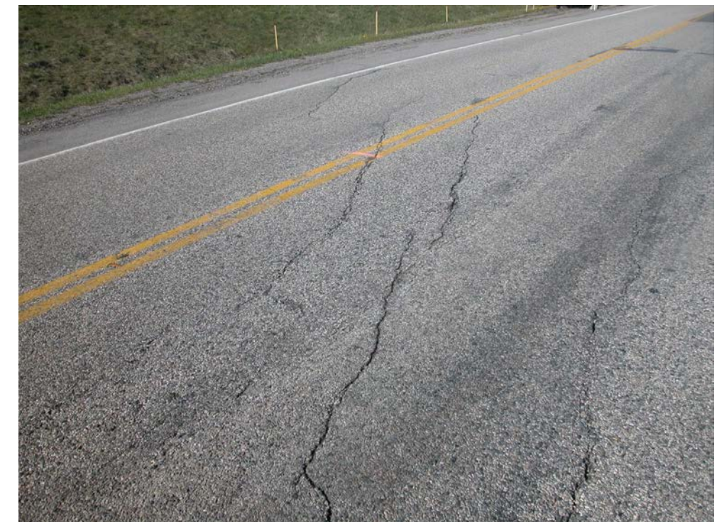
Photo S2-3 (lower left) – May 2004 – closer view of the bend in the guardrail at the east end of the site. Also note the cracking visible around the yellow centerline of the road on the left side of the photo – this cracking was also noted during the July 2003 inspection and has not changed significantly since that time. This cracking may delineate the east flank of road disturbance due to slope movement at this site.
