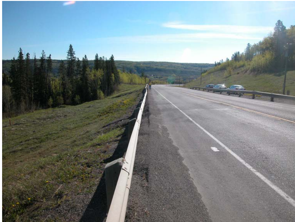
Photo S2-1 (upper left) – May 2004 – facing east across the S2-Priddis site. Note the slight bend in the guardrail visible at the far (east) end. The landslide area is visible on the slope below the road, on the left side of the photo. Photo S2-5 shows another view of the landslide area.
