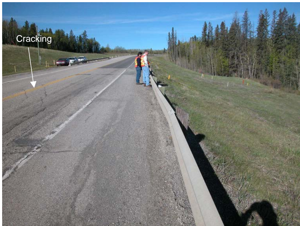
Photo S2-3 (lower left) – May 2004 – closer view of the bend in the guardrail at the east end of the site. Also note the cracking visible around the yellow centerline of the road on the left side of the photo – this cracking was also noted during the July 2003 inspection and has not changed significantly since that time. This cracking may delineate the east flank of road disturbance due to slope movement at this site.
