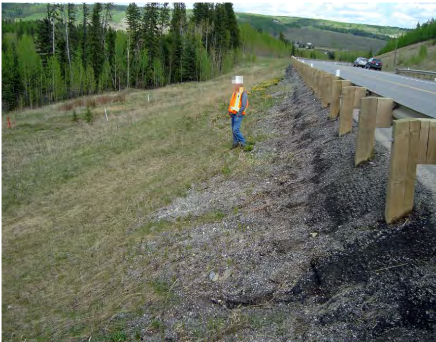
Photo S2-3 (May 2013) – Facing eastbound along the downslope shoulder of the highway from the west end of the landslide area.
