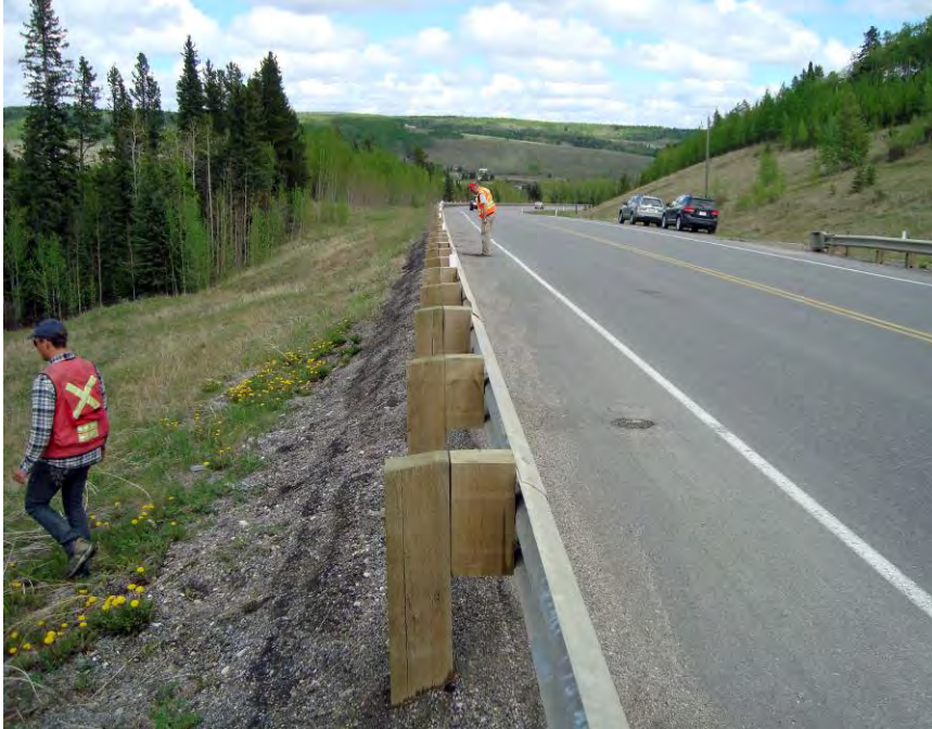
Photo S2-2 (May 2013) – Facing eastbound along the pile wall area.
