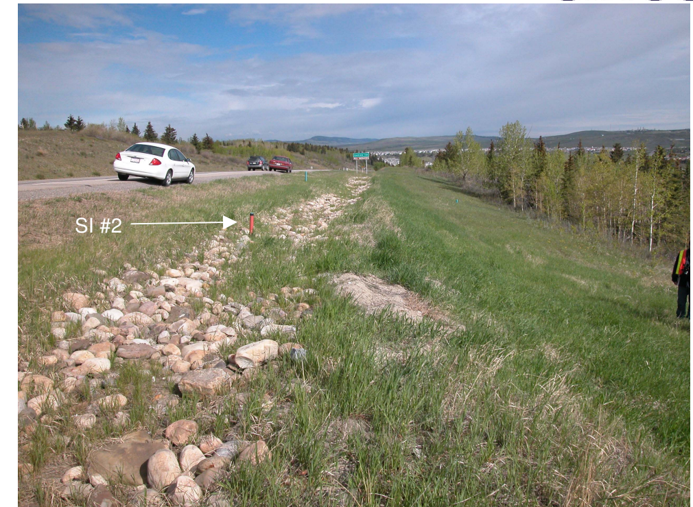
Photo S3-4 (upper left) – May 2004 – facing west along the north shoulder of the highway at S3 – Cochrane. The ditch appears to be functioning well although the low area in the downslope berm between SI #2 and SI #5 noted in previous inspections should be repaired to restore the overall ditch gradient and capacity and convey surface runoff away from this site.
