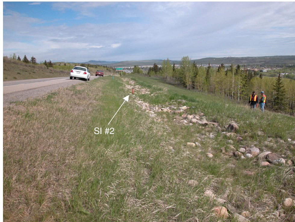
Photo S3-4 (upper left) – May 2004 – facing west along the north shoulder of the highway at S3 – Cochrane. The ditch appears to be functioning well although the low area in the downslope berm between SI #2 and SI #5 noted in previous inspections should be repaired to restore the overall ditch gradient and capacity and convey surface runoff away from this site.
