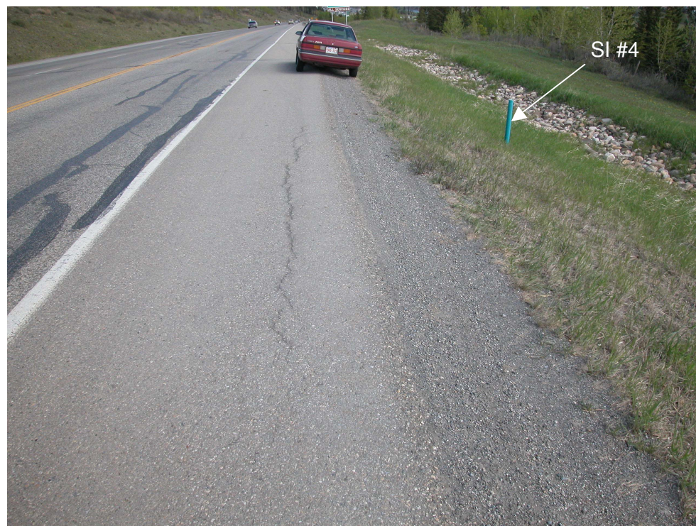
Photo S3-6 (lower left) – May 2004 – crack in the road near SI #4 – no significant change since the July 2003 inspection.
