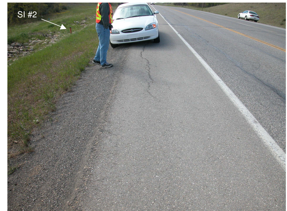
Photo S3-6 (lower left) – May 2004 – crack in the road near SI #4 – no significant change since the July 2003 inspection.
