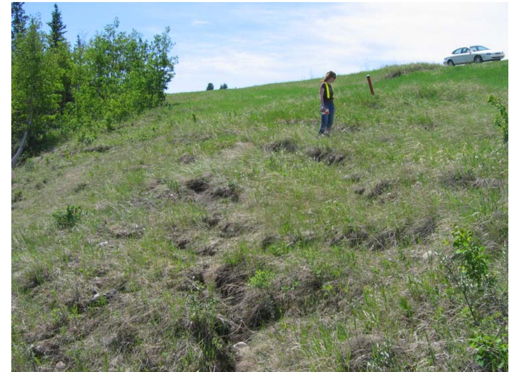
Photo S3-7 (lower right) – June 2006 – shallow sloughing on slope to the north of the road.
