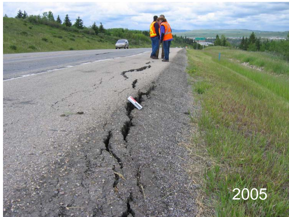
Photo S3-3 (lower left) – June 2005 – facing west along the road. Large cracks in the shoulder developed between the time May 2005 instrument readings and the late June 2005 annual site inspection.
