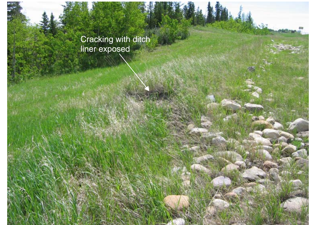
Photo S3-3 (lower left) – June 2005 – facing west along the road. Large cracks in the shoulder developed between the time May 2005 instrument readings and the late June 2005 annual site inspection.
