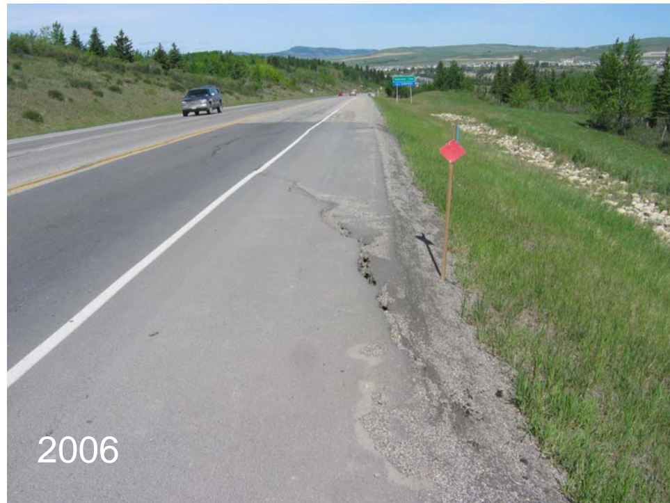
Photo S3-1 (upper left) – June 2006 – facing west along the road. Large cracks in the shoulder redeveloped after being repaired in the summer of 2005.
