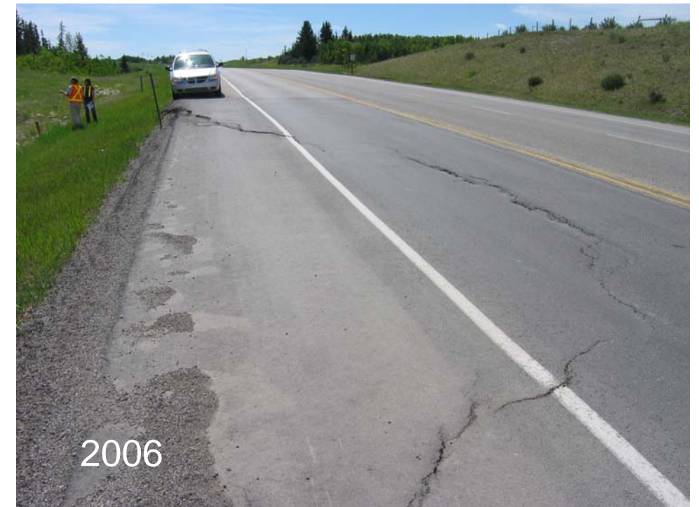
Photo S3-1 (upper left) – June 2006 – facing west along the road. Large cracks in the shoulder redeveloped after being repaired in the summer of 2005.
