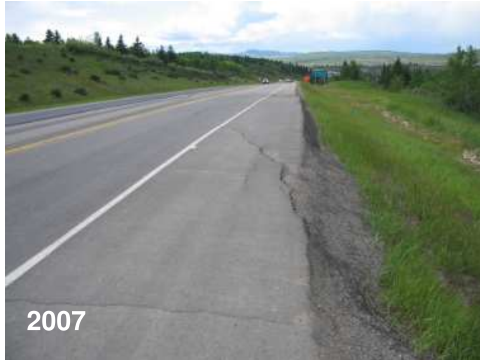
Photo S3-1 – June 2007 (upper left) Facing west along the road with cracking and downdrop of the pavement along the shoulder and in the northbound lane visible. The pattern of the cracking appears to form a circular landslide headscarp that has retrogressed into the northbound lane of the highway.
