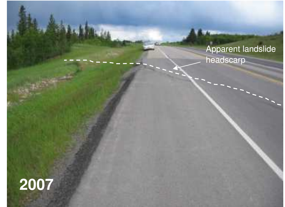
Photo S3-1 – June 2007 (upper left) Facing west along the road with cracking and downdrop of the pavement along the shoulder and in the northbound lane visible. The pattern of the cracking appears to form a circular landslide headscarp that has retrogressed into the northbound lane of the highway.
