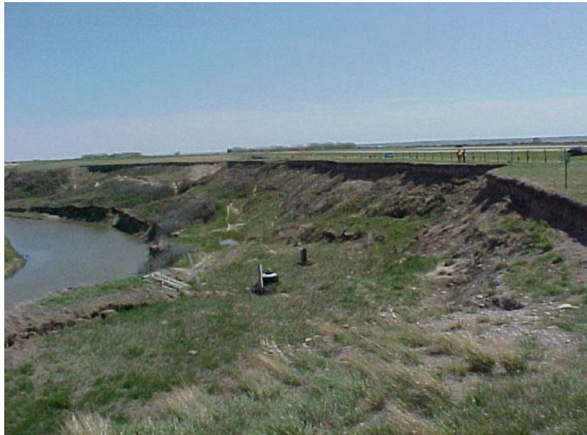
Photo 7 – Facing south across slide area. Note river erosion at toe of slide.
