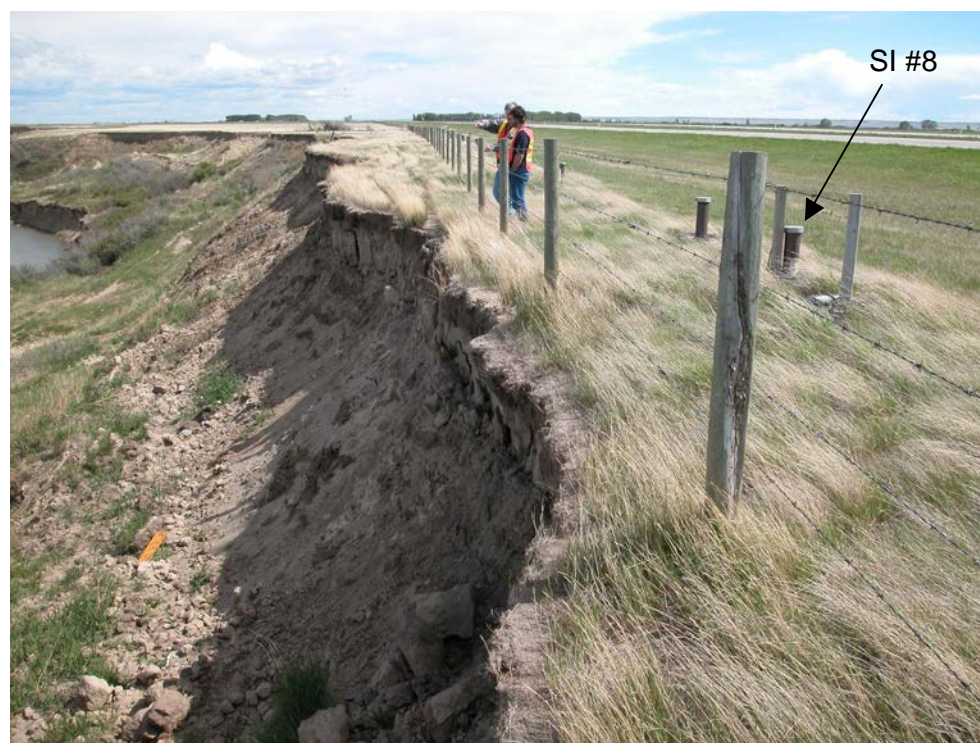
Photo S4-2 (upper right) – May 2004 – facing south towards the point of maximum crest retrogression relative to the fenceline.
