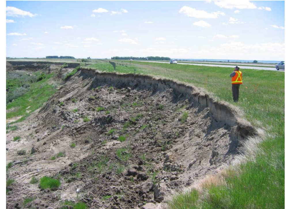
Photo S4-1 (upper left) – May 2006 – facing north across the area where the landslide scarp has retrogressed further past the fenceline and towards the road since the 2005 inspection.
