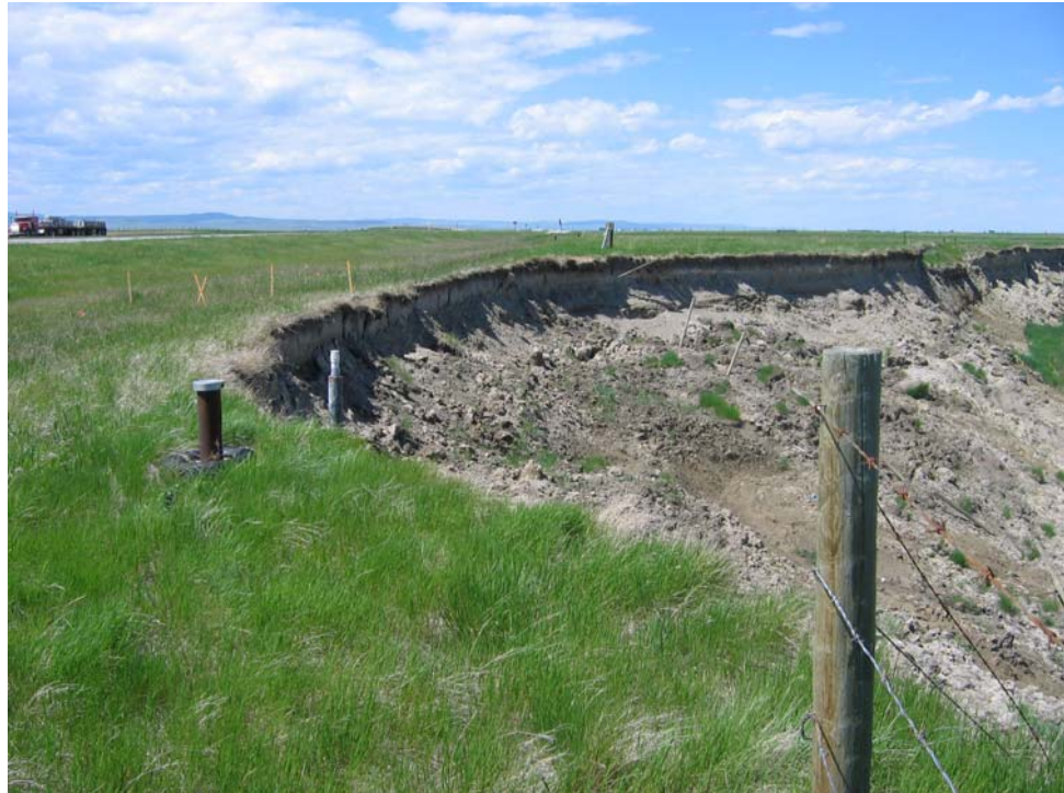
Photo S4-1 (upper left) – May 2006 – facing north across the area where the landslide scarp has retrogressed further past the fenceline and towards the road since the 2005 inspection.
