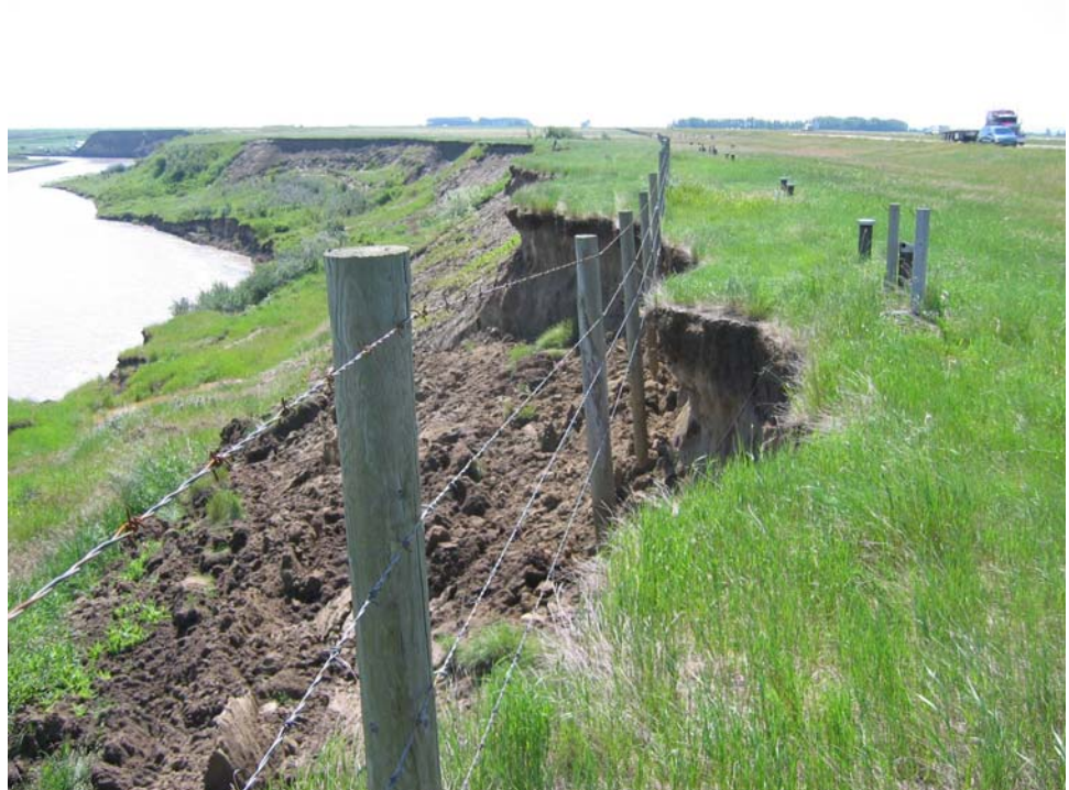
Photo S4-3 (lower left) – June 2005 – point of maximum slope crest retrogression towards the road as of June 2005.
