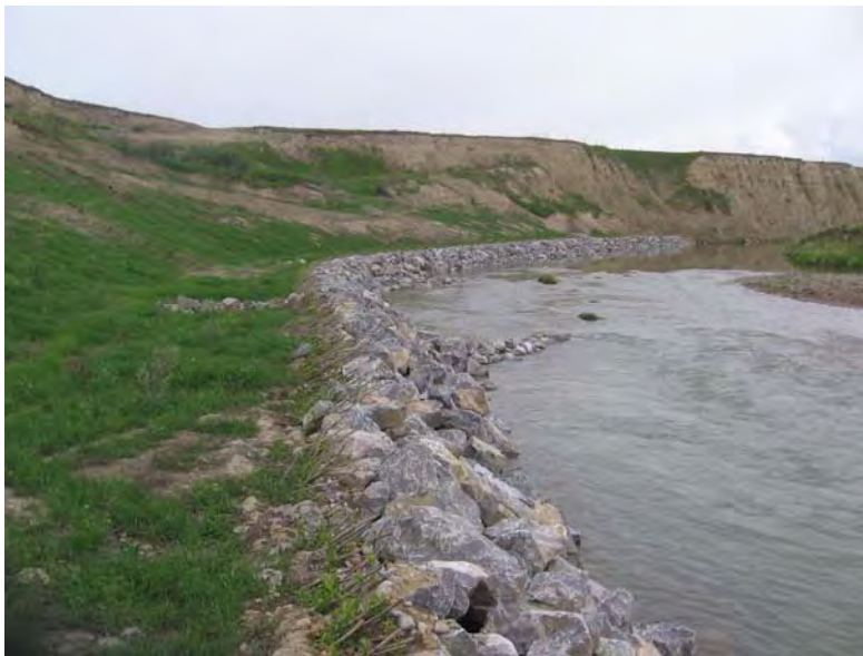
Photo S4-2 (bottom) – June 2009 Facing upstream along the LPSTP along the right creek bank, with the rocks vanes angling into the channel visible.
