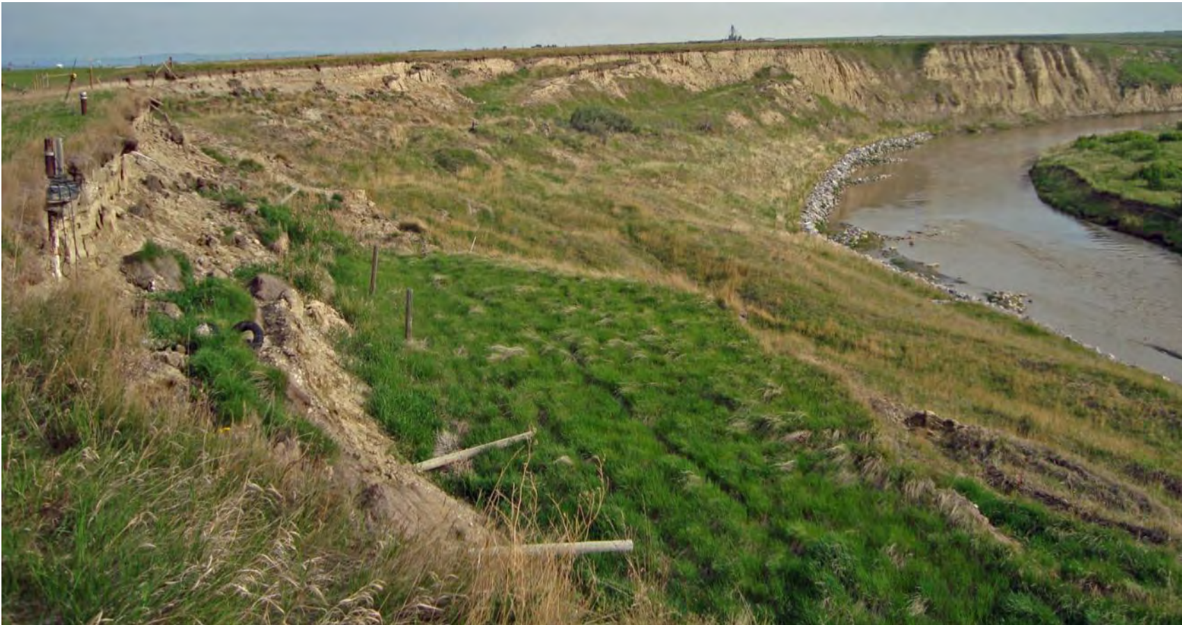
Photo S4-5 (May 2013) – Facing north at the slide area with a view of the lower slope and river bank. Note the sedimentation within the vanes and the improved vegetation cover.
