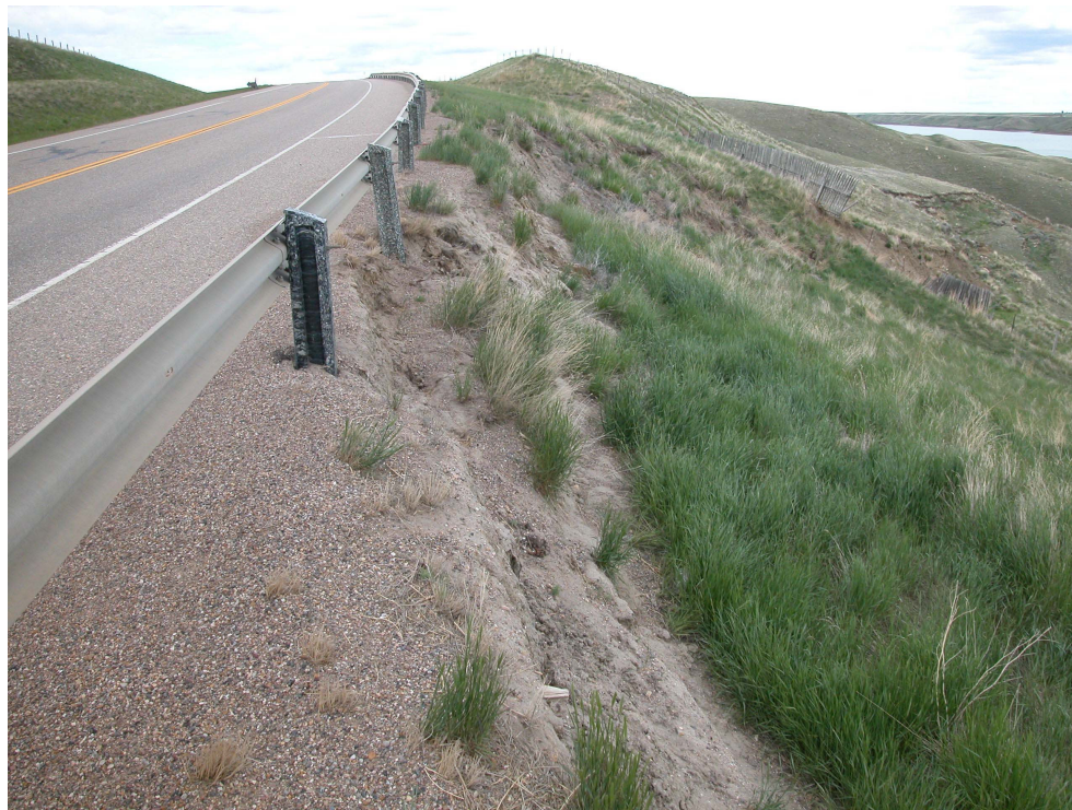
Photo S5-1 (upper left) – May 2004 – facing east across the shallow slumping area immediately downslope of the guardrail along the downslope edge of the road. The slumping has undermined some of the guardrail posts. It does not appear that significant additional movement has occurred since the July 2003 inspection, however the potential for additional movement in response to precipitation and surface runoff remains.
