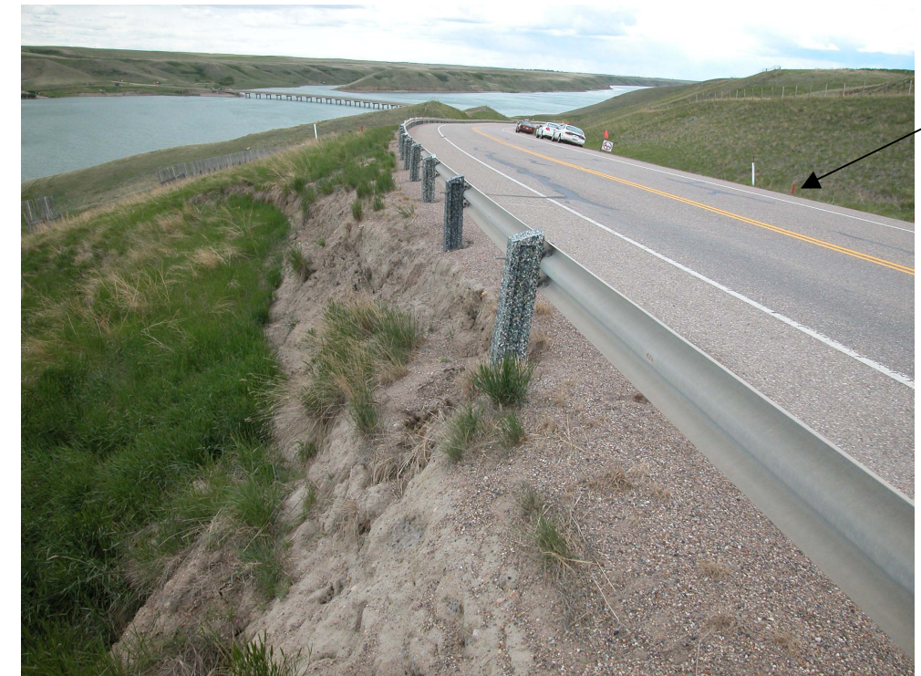
Photo S5-1 (upper left) – May 2004 – facing east across the shallow slumping area immediately downslope of the guardrail along the downslope edge of the road. The slumping has undermined some of the guardrail posts. It does not appear that significant additional movement has occurred since the July 2003 inspection, however the potential for additional movement in response to precipitation and surface runoff remains.
