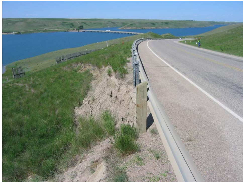
Photo S5-3 (lower left) – May 2006 – facing west across the shallow slumping area below the road. The guardrail posts are becoming undermined, but the shallow slumping has not yet retrogressed into the paved road surface.
