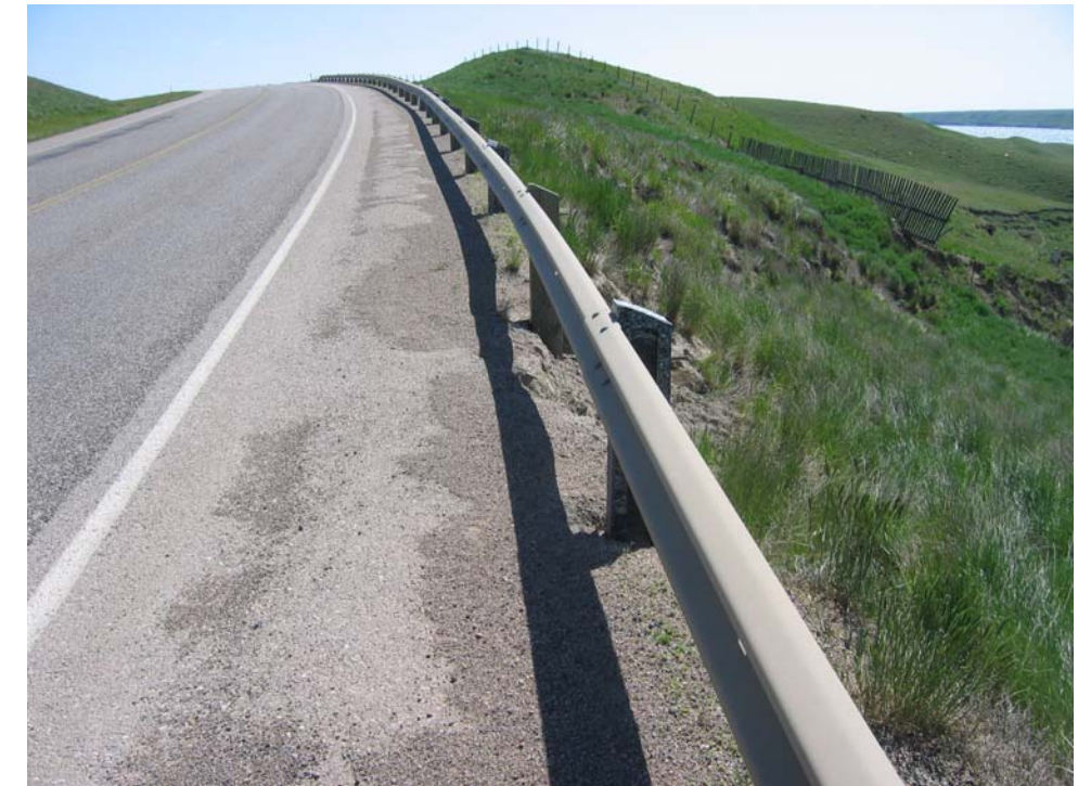
Photo S5-3 (lower left) – May 2006 – facing west across the shallow slumping area below the road. The guardrail posts are becoming undermined, but the shallow slumping has not yet retrogressed into the paved road surface.
