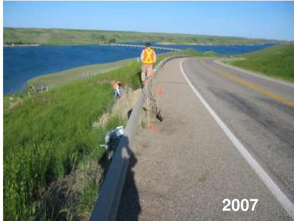
Photo S5-1 – June 2007 (upper left) Facing west across the shallow slumping area below the road. The shallow slumping has started to retrogress into the paved road surface since the May 2006 site inspection. Compare with Photo S5-2 which shows the same area as seen during the May 2006 site inspection.
