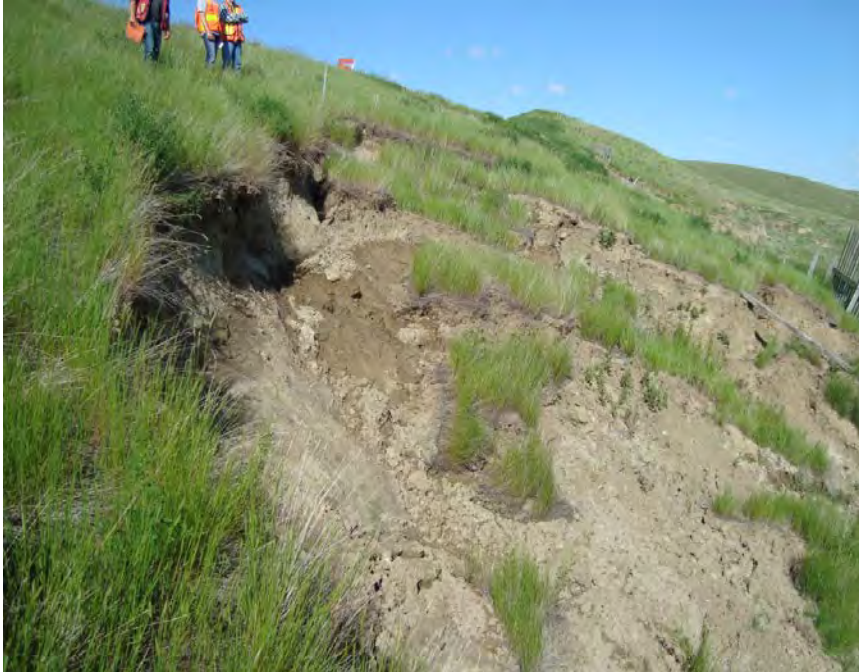
Photo S5-4 (June 2011) – An active scarp at the west slide flank noted during the 2011 inspection. Refer to Photo S5-5 for comparison from the 2013 inspection.
