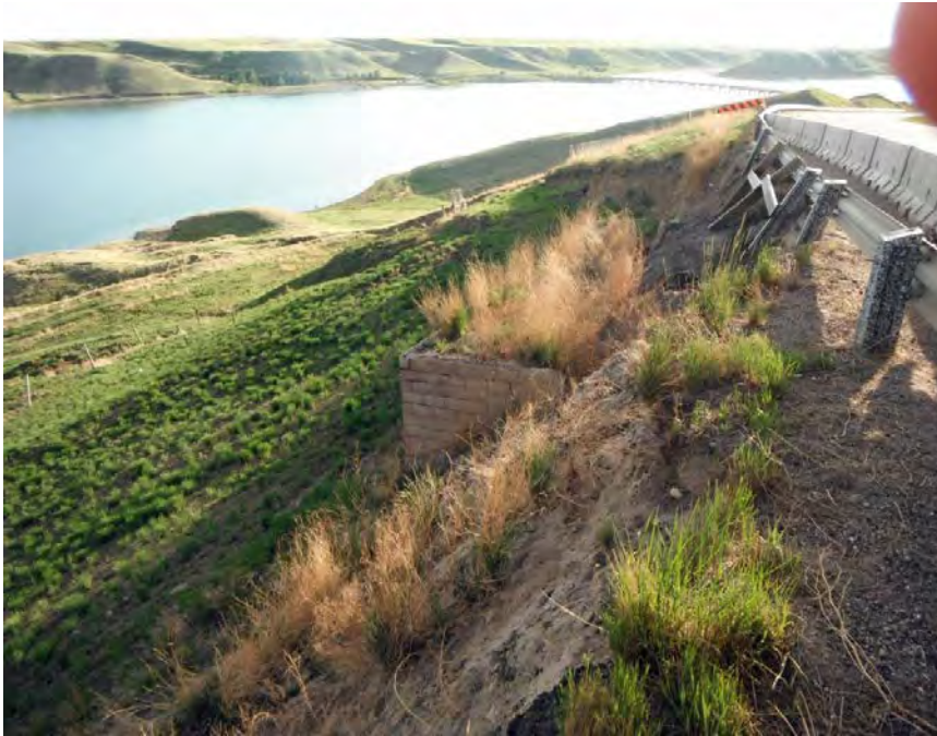
Photo S5-3 (May 2013) – Standing on the south road shoulder looking towards the southwest at the headscarp retrogression into the road surface and retaining wall.
