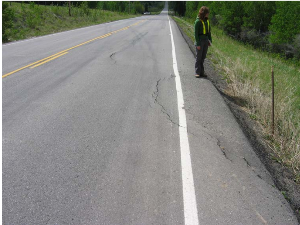
Photo S8-1 (upper left) – May 2006 – facing south along the northern area of the site. New cracking observed in the previously-noted cracking and settlement area. The visible cracking has developed since the area was repaved after the 2005 inspection.
