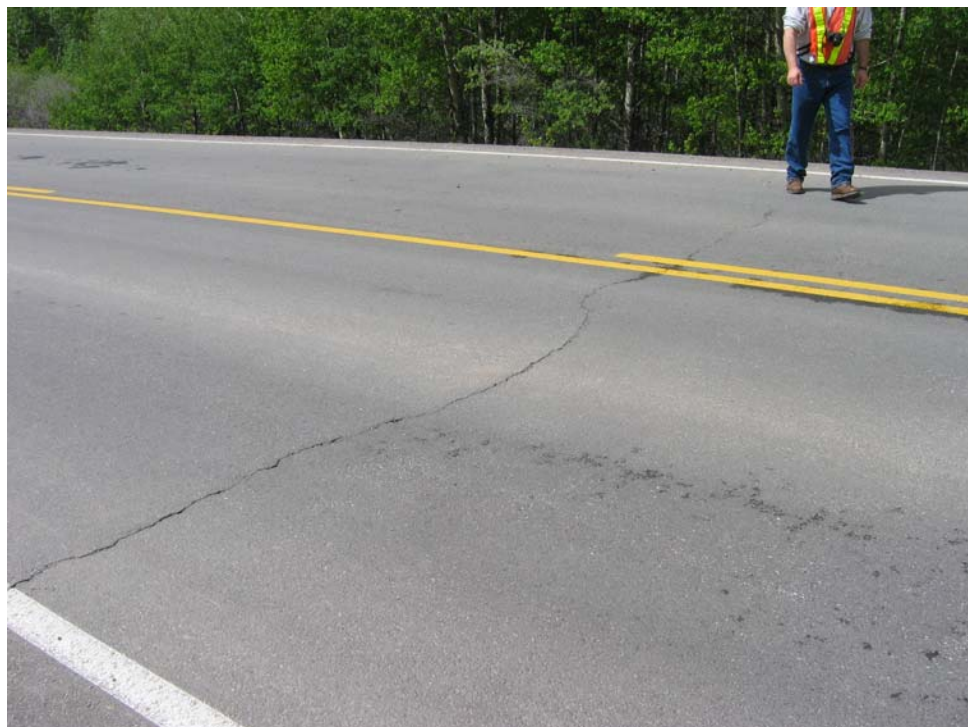
Photo S8-3 (lower left) – May 2006 – new crack in the road surface approximately 12 m south of the estimated north edge of the area that was repaved since the June 2005 inspection.
