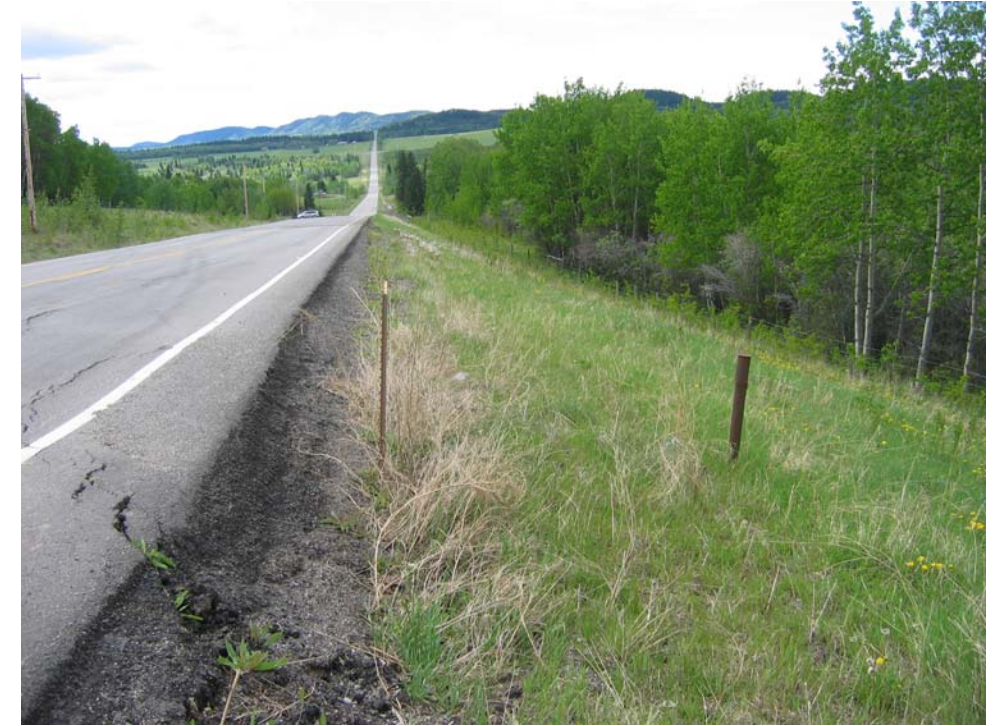
Photo S8-1 (upper left) – May 2006 – facing south along the northern area of the site. New cracking observed in the previously-noted cracking and settlement area. The visible cracking has developed since the area was repaved after the 2005 inspection.
