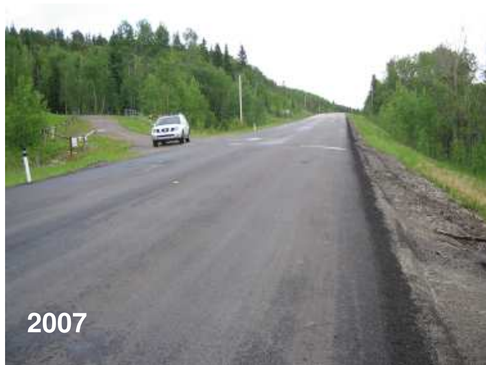
Photo S10(A)-3 – June 2007 (lower left) Facing south across the site.
