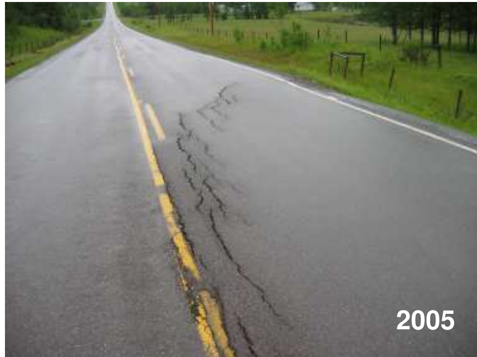
Photo S10(C)-1 – June 2005 (upper left) Cracking and settlement of the road surface as observed during the 2005 site inspection.
