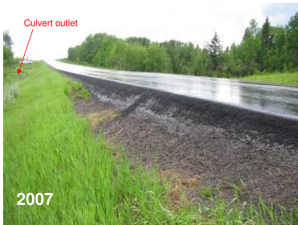
Photo S10(C)-3 – June 2007 (lower left) Closer view of the edge of the recent overlay, along the east shoulder of the road. The approximate location of the culvert to the south of the overlay is shown.
