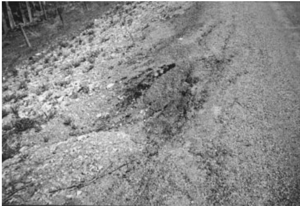
Photo 2 – Site A shoulder of highway.
