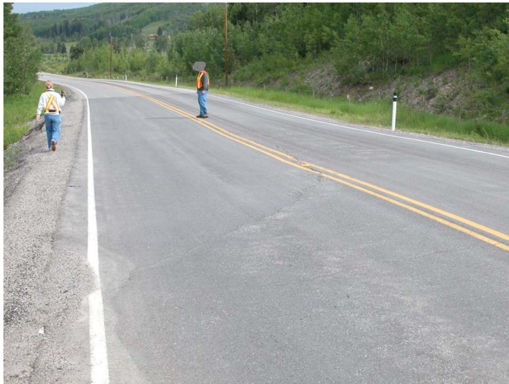
Photo 1 (upper left) Site A Facing north across the area that has been patched since the May 2002 site inspection. Compare the cracking pattern with Photo 2 – the same movement is ongoing.
