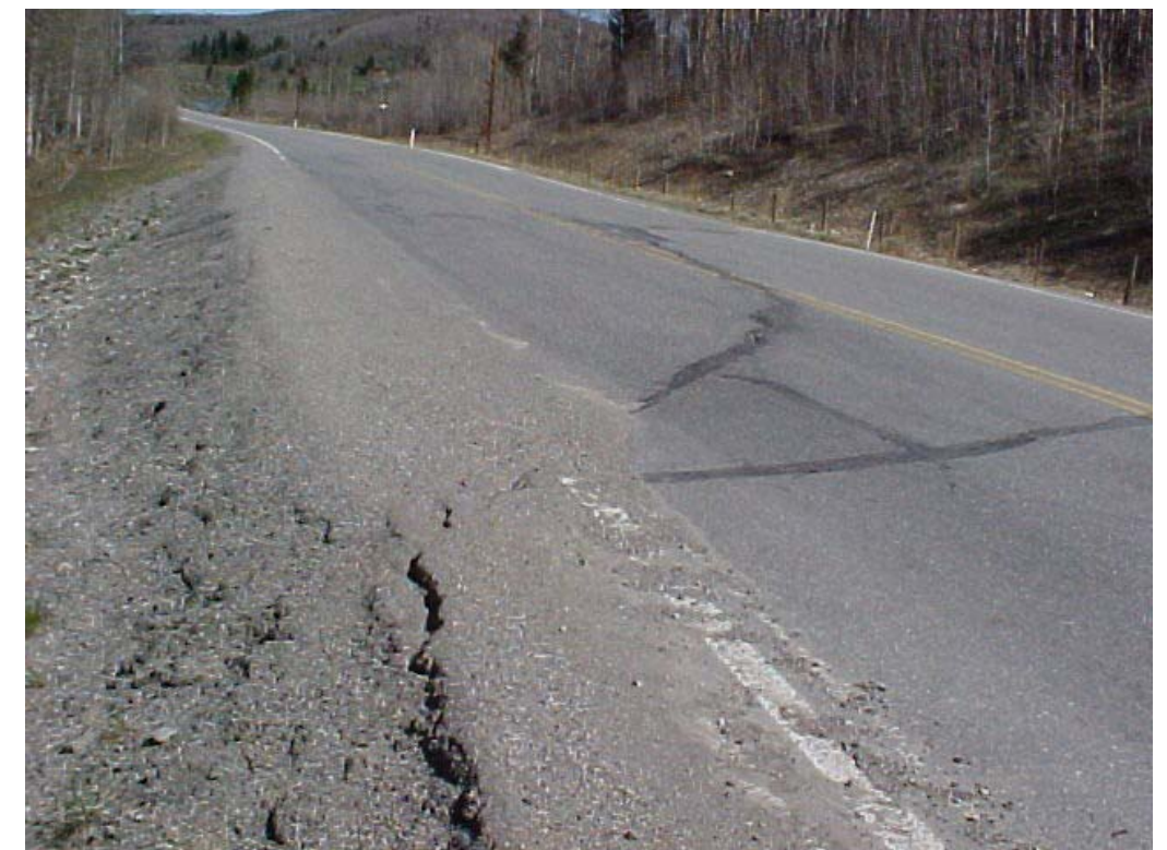
Photo 1 (upper left) Site A Facing north across the area that has been patched since the May 2002 site inspection. Compare the cracking pattern with Photo 2 – the same movement is ongoing.
