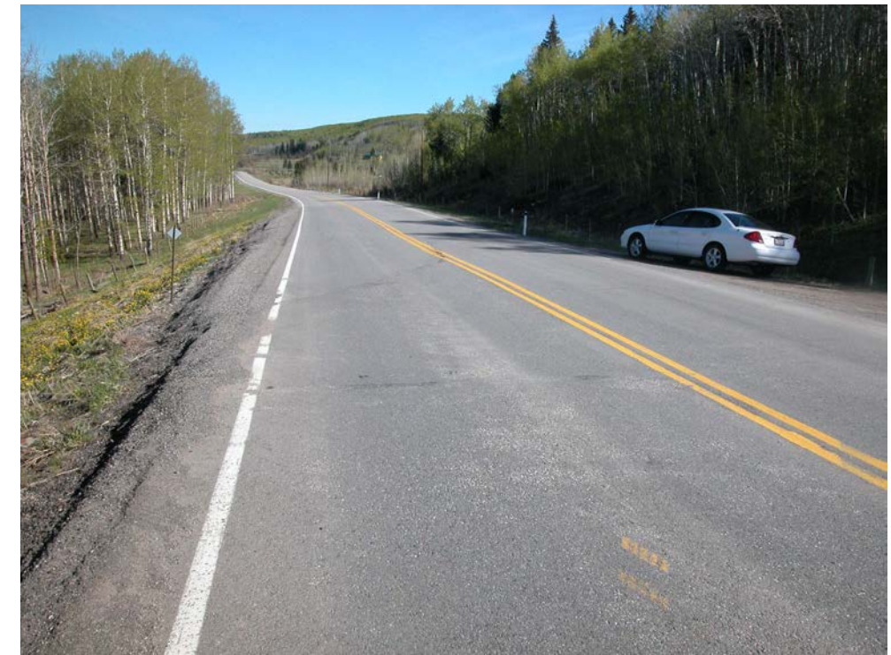
Photo S10A-2 (upper right) – May 2004 – wider view of the area shown in Photo S10A-1. The shape of the affected area suggests a slump downwards to the west (left).
