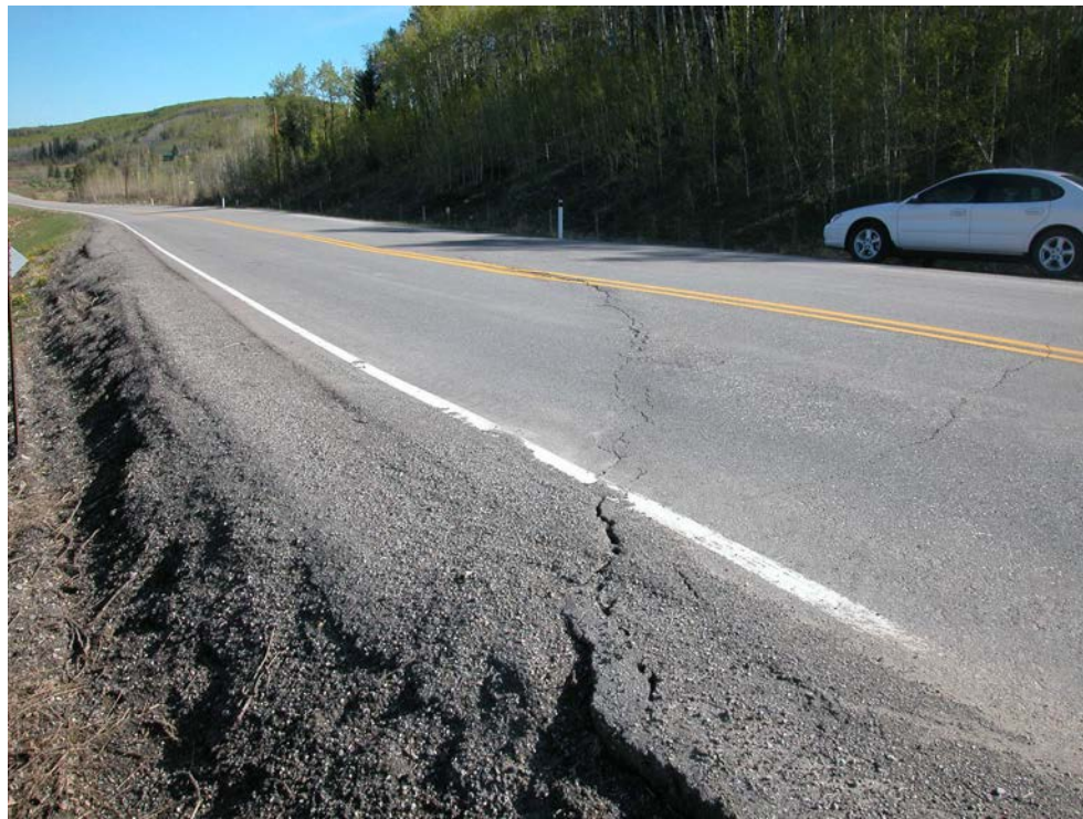
Photo S10A-3 (lower left) – May 2004 – facing south across the settlement and cracking area shown in Photos S10A-1 and S10A-2. The north flank of the cracking is visible in the lower left corner of the photo and the south flank is visible in the middle background. The segment of the road surface between the edges of the cracking measures approximately 30 m along the west (right) shoulder of the road.
