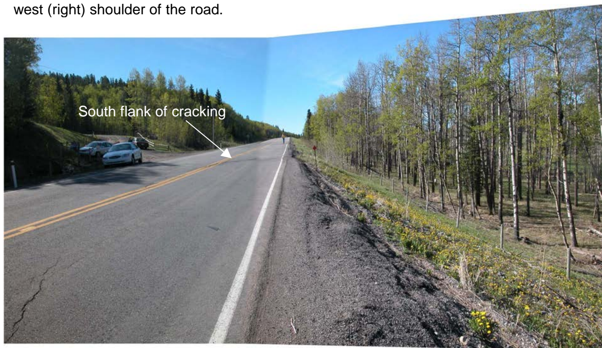
Photo S10A-4 (lower right) – May 2004 – possible secondary cracking in the southbound lane, approximately 15 m south of the south flank of the main cracking area shown in Photos S10A-1 to S10A-3.
