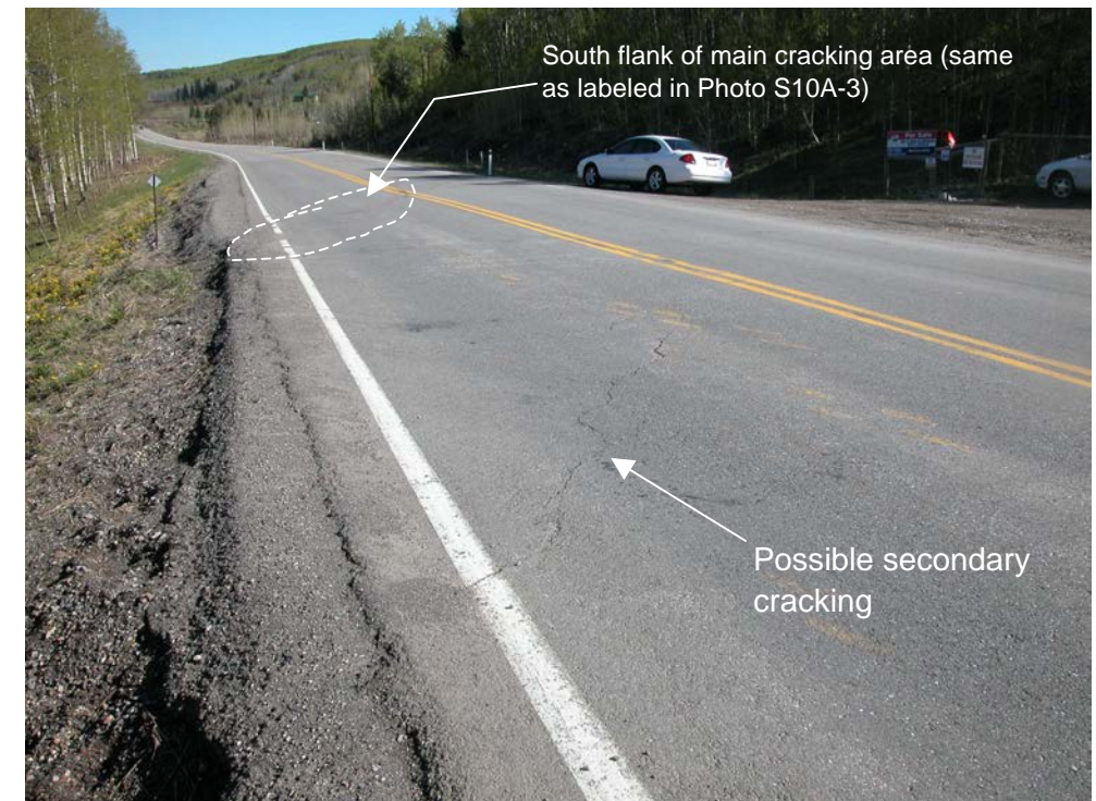
Photo S10A-4 (lower right) – May 2004 – possible secondary cracking in the southbound lane, approximately 15 m south of the south flank of the main cracking area shown in Photos S10A-1 to S10A-3.
