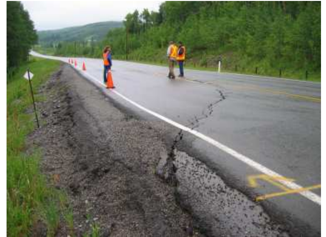
Photo S10(A)-1 (upper left) – June 2005 – facing north across the settlement and cracking area in the southbound lane. This area was repaved in 2004 and the current cracking is in the same location and pattern noted in previous years.
