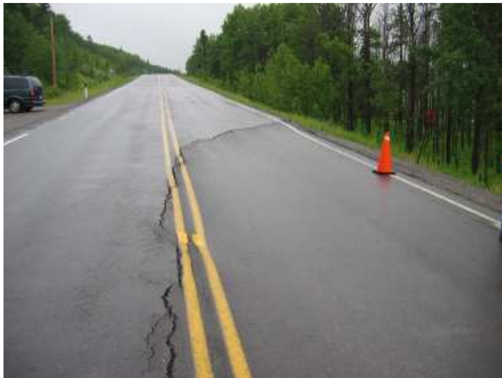
Photo S10(A)-3 (lower left) – June 2005 – facing south across site S10(A). The southbound lane has settled up to approximately 100 mm, apparently mostly during and after the heavy rains in June 2005.
