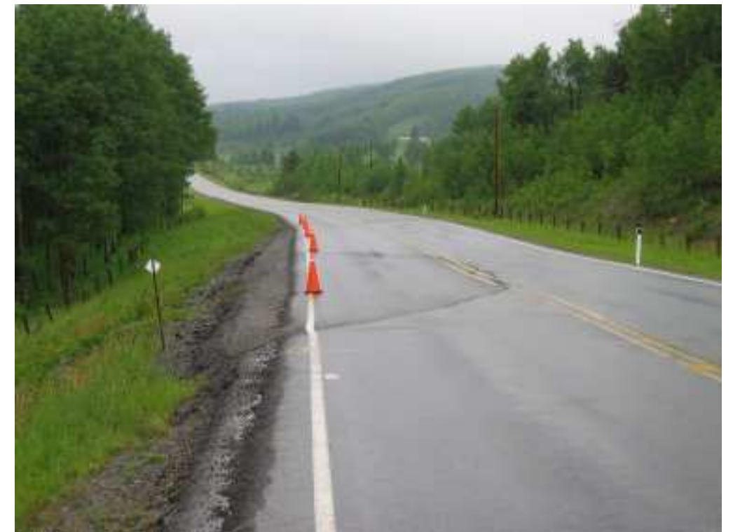
Photo S10(A)-3 (lower left) – June 2005 – facing south across site S10(A). The southbound lane has settled up to approximately 100 mm, apparently mostly during and after the heavy rains in June 2005.
