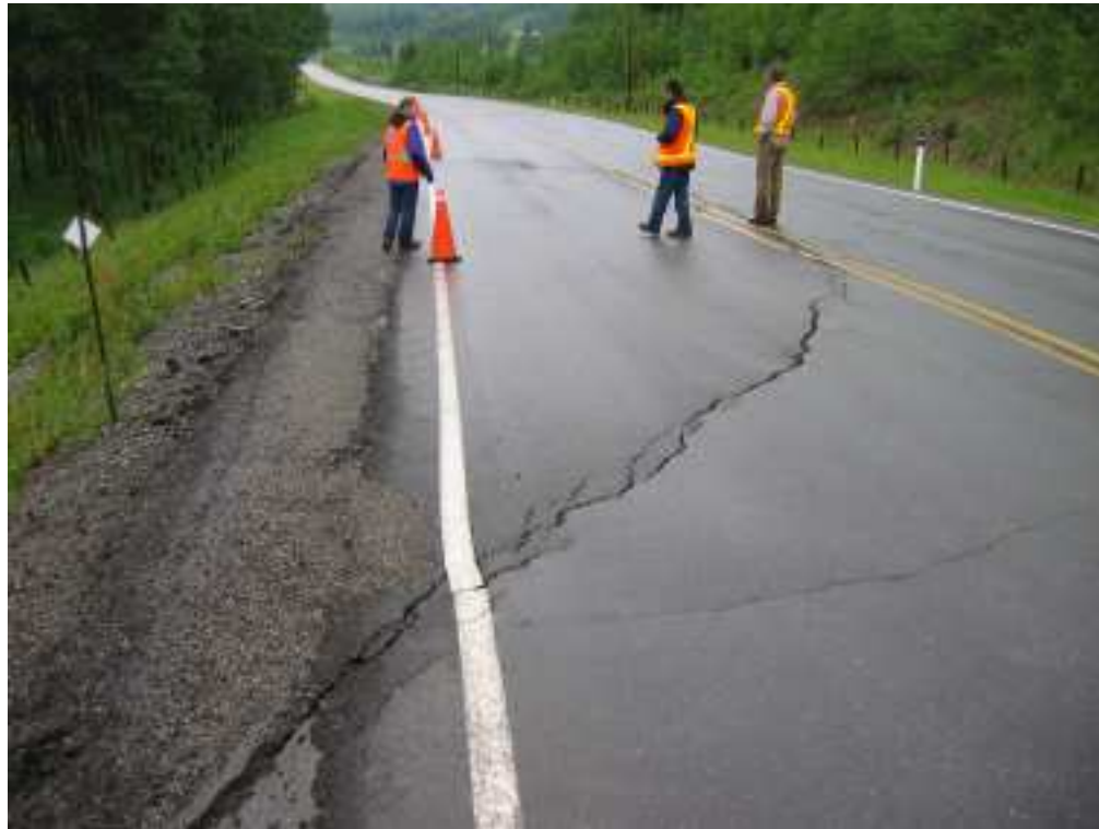
Photo S10(A)-1 (upper left) – June 2005 – facing north across the settlement and cracking area in the southbound lane. This area was repaved in 2004 and the current cracking is in the same location and pattern noted in previous years.
