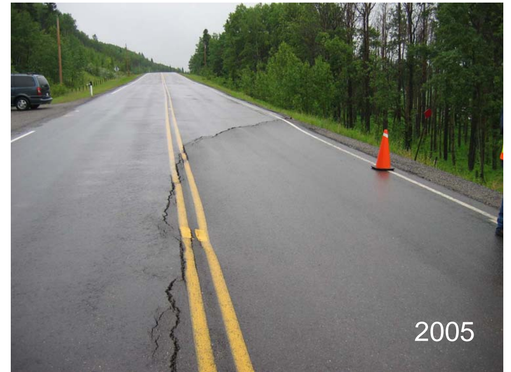
Photo S10(A)-3 (lower left) – June 2005 – facing north across the settlement and cracking area observed at the time of the 2005 site inspection. The pattern of damage to the road surface suggests a slump failure down towards the west (left on the photo).
