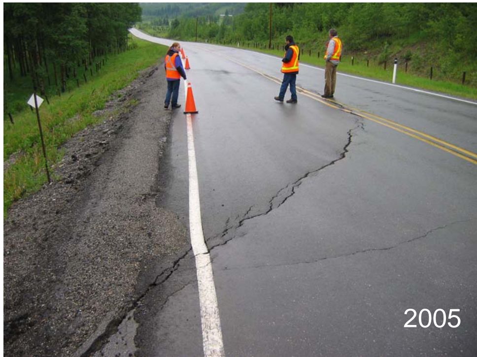
Photo S10(A)-3 (lower left) – June 2005 – facing north across the settlement and cracking area observed at the time of the 2005 site inspection. The pattern of damage to the road surface suggests a slump failure down towards the west (left on the photo).
