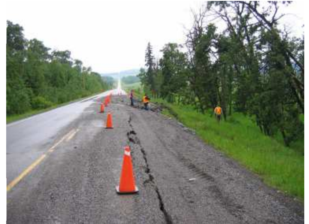
Photo S10(B)-1 (upper left) – June 2005 – facing south across the portion of the southbound lane damaged by the instability caused by heavy rainfall in June 2005.
