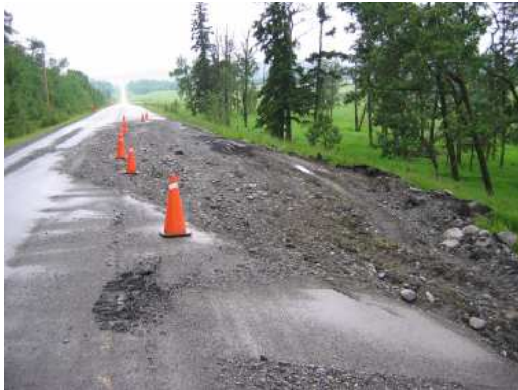
Photo S10(B)-1 (upper left) – June 2005 – facing south across the portion of the southbound lane damaged by the instability caused by heavy rainfall in June 2005.
