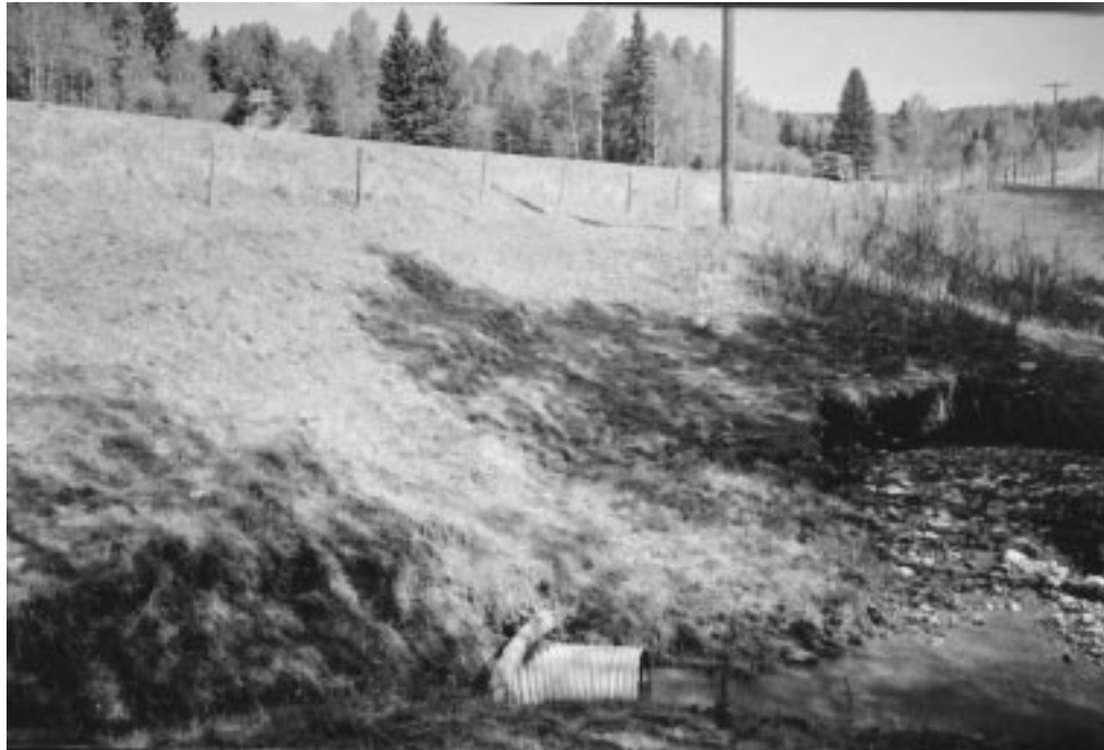
Photo 7 –Site C – Downstream (east) side of embankment (looking north).
