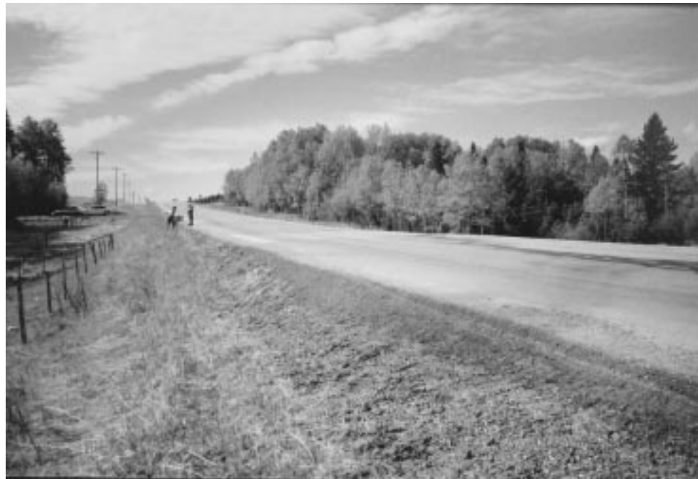
Photo 6 –Site C – Showing dip in highway.
