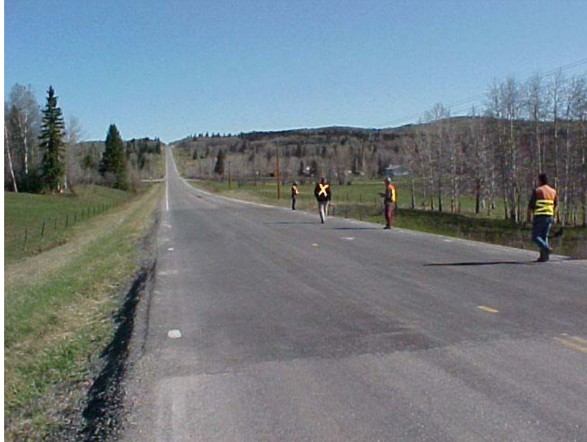
Photo 9 – Site C – facing north (May 2002).
