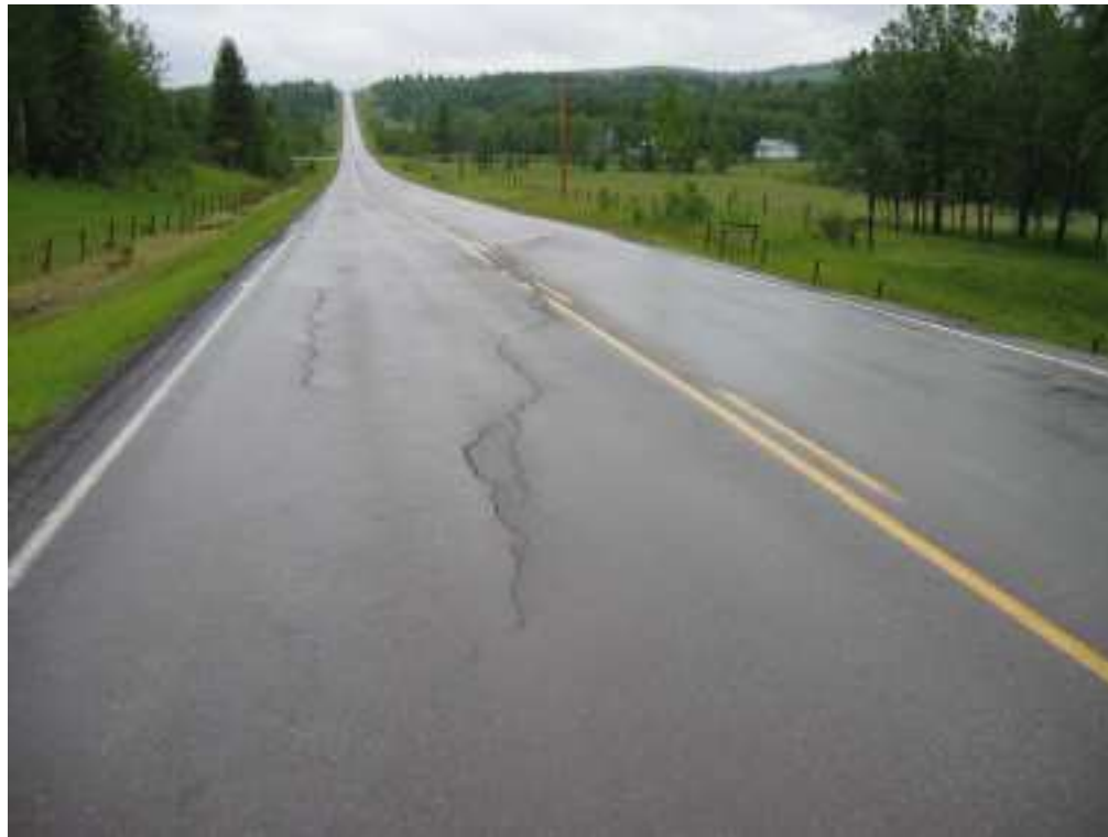
Photo S10(C)-1 (upper left) – June 2005 – facing north across recent cracking that extends in an arc from the east shoulder to the southbound lane. The center of the cracking is approximately 45 m north of the culvert below the road.
