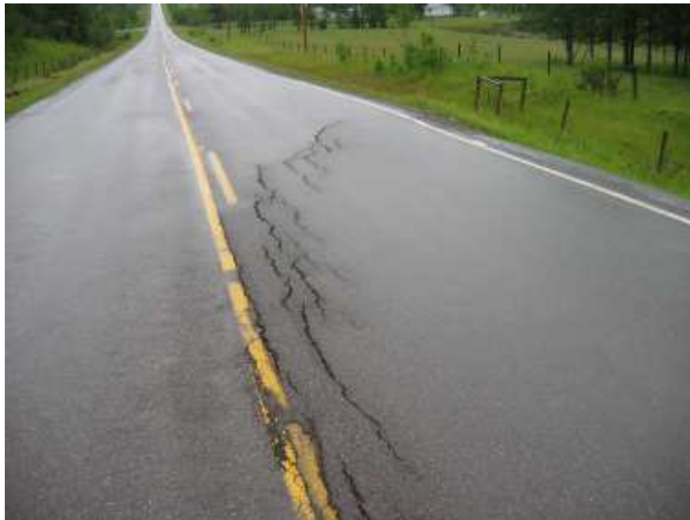
Photo S10(C)-3 (lower left) – June 2005 – closer view of the north end of the cracking and settlement in the southbound lane.
