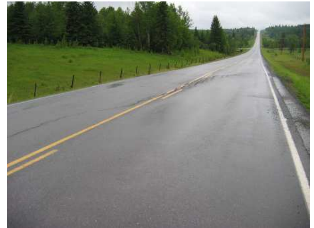
Photo S10(C)-1 (upper left) – June 2005 – facing north across recent cracking that extends in an arc from the east shoulder to the southbound lane. The center of the cracking is approximately 45 m north of the culvert below the road.
