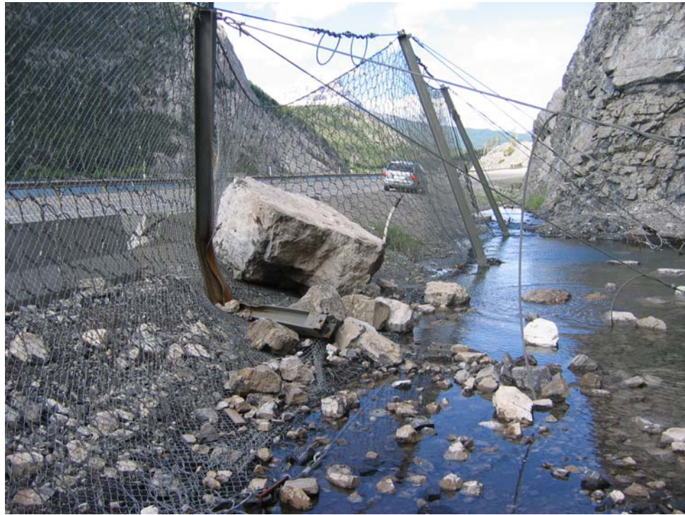
Photo S15-1 (upper left) – May 2006 – boulder from April 2006 rockfall event that struck and destroyed one of the support posts but was retained by the barrier.
