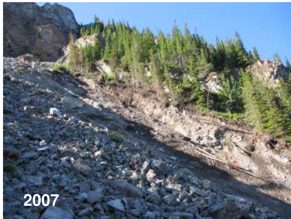
Photo S15-6 – June 2007 (lower left) The gully headwall on the slope above the barrier net. This headwall has eroded and expanded in recent years. Compare with Photo S15-7 that shows the same area as it appeared in September 2003.
