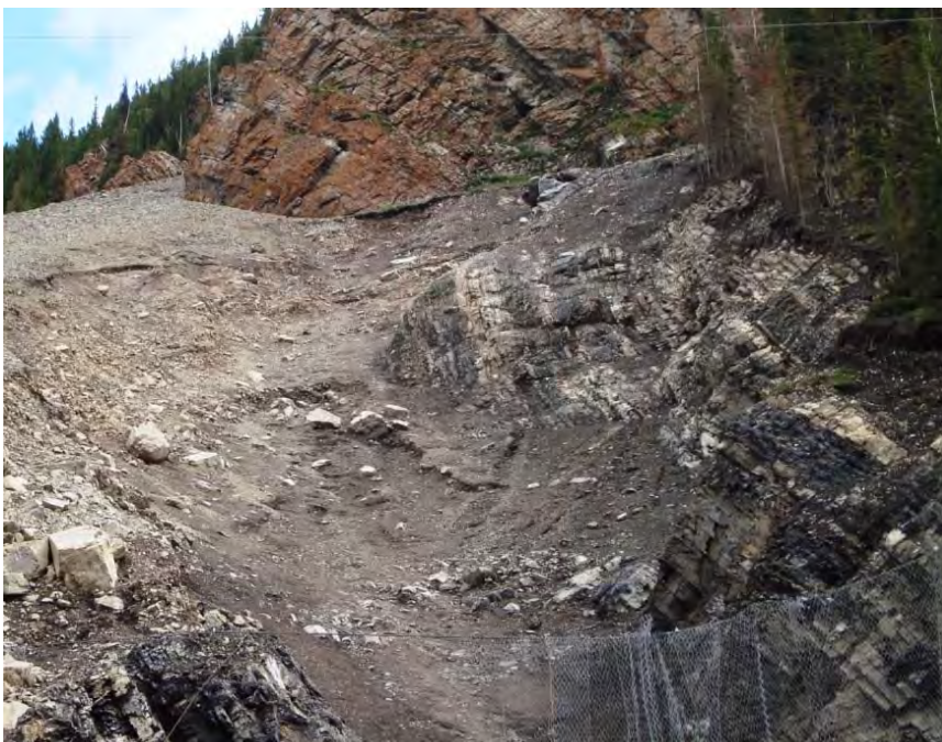
Photo S15-4 (June 2012) – The upper gully in the talus slope as observed during the 2012 inspection. It continues to expand toward the cliff face as it appears to have slightly retrogressed since 2011.
