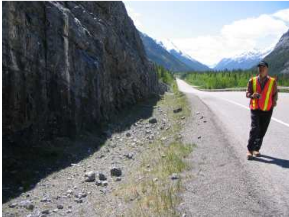
Photo S18-4 – June 2007 (upper left) Facing southbound along the east edge of Highway 40 in the southern/central portion of the East Cut Slope. Note the accumulation of rockfall debris in the ditch and the proximity of some of the rocks to the east edge of the pavement.
