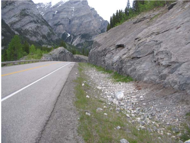
Photo S18-1 (top) – June 2008 Facing northbound along the east highway ditch from the south end of the site. The ditch is of sufficient size in this area to keep the rockfall debris from the East Cut Slope from impacting the road.
