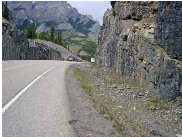
Photo S18-4 – June 2009 Facing northbound along the east ditch south of the centre of the rock cut. Minor rockfall in this area has not likely landed on the road.
