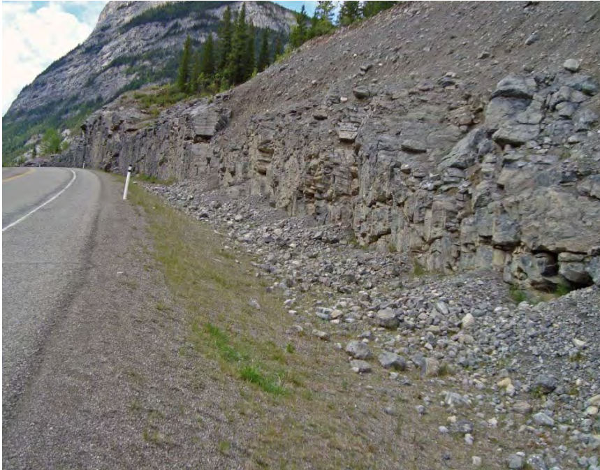
Photo S18-4 – June 2012 Facing southbound along the west ditch. All rock fall is contained within the ditch.
