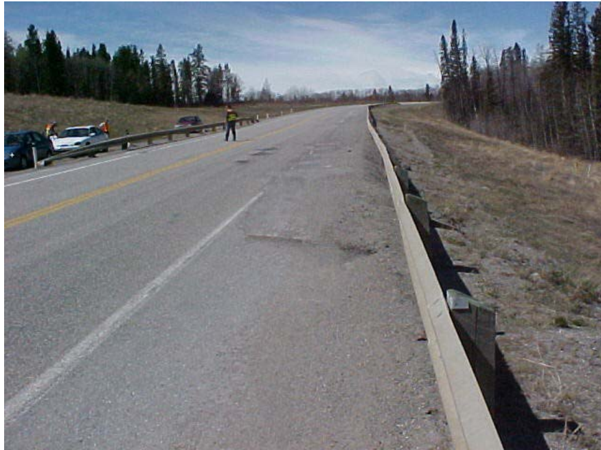
Photo 1 – Facing west along the downslope edge of the road through the slide area. The existing pile wall is located just to the left of the guardrail. Note how the guardrail has been displaced by settlement of the road, and the loss of ground downslope of the guardrail.
