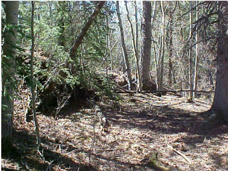
Photo 3 – May 2002 photo of toe of slide approximately 150 m below road.
